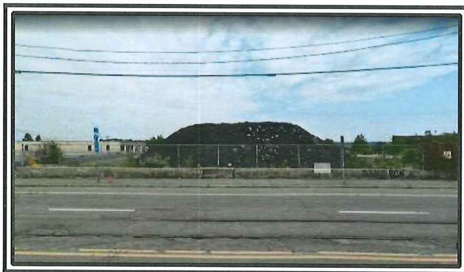
Asphalt Area from Allens Ave (2019 Google Streetview)
