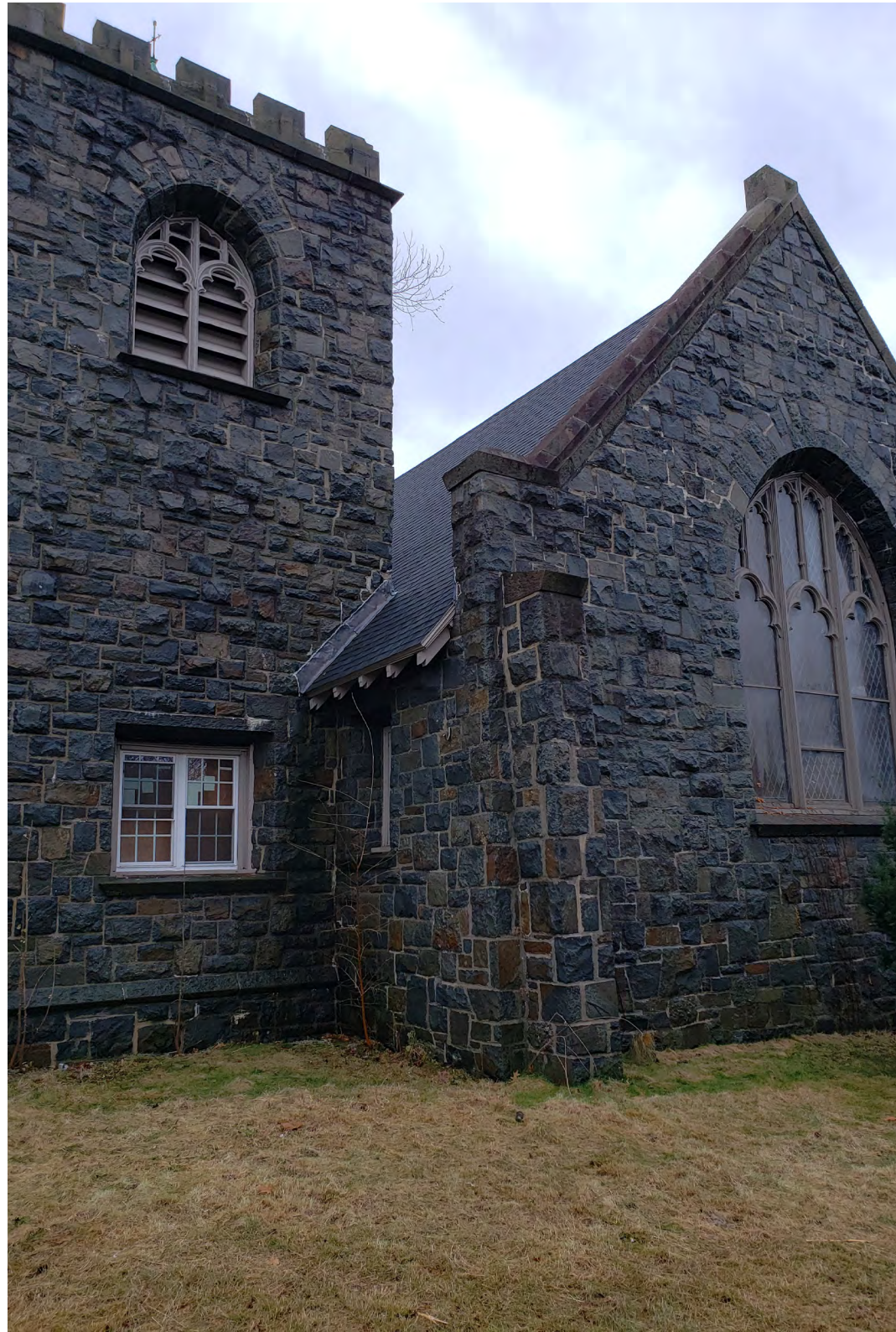
VIEW OF TOWER
