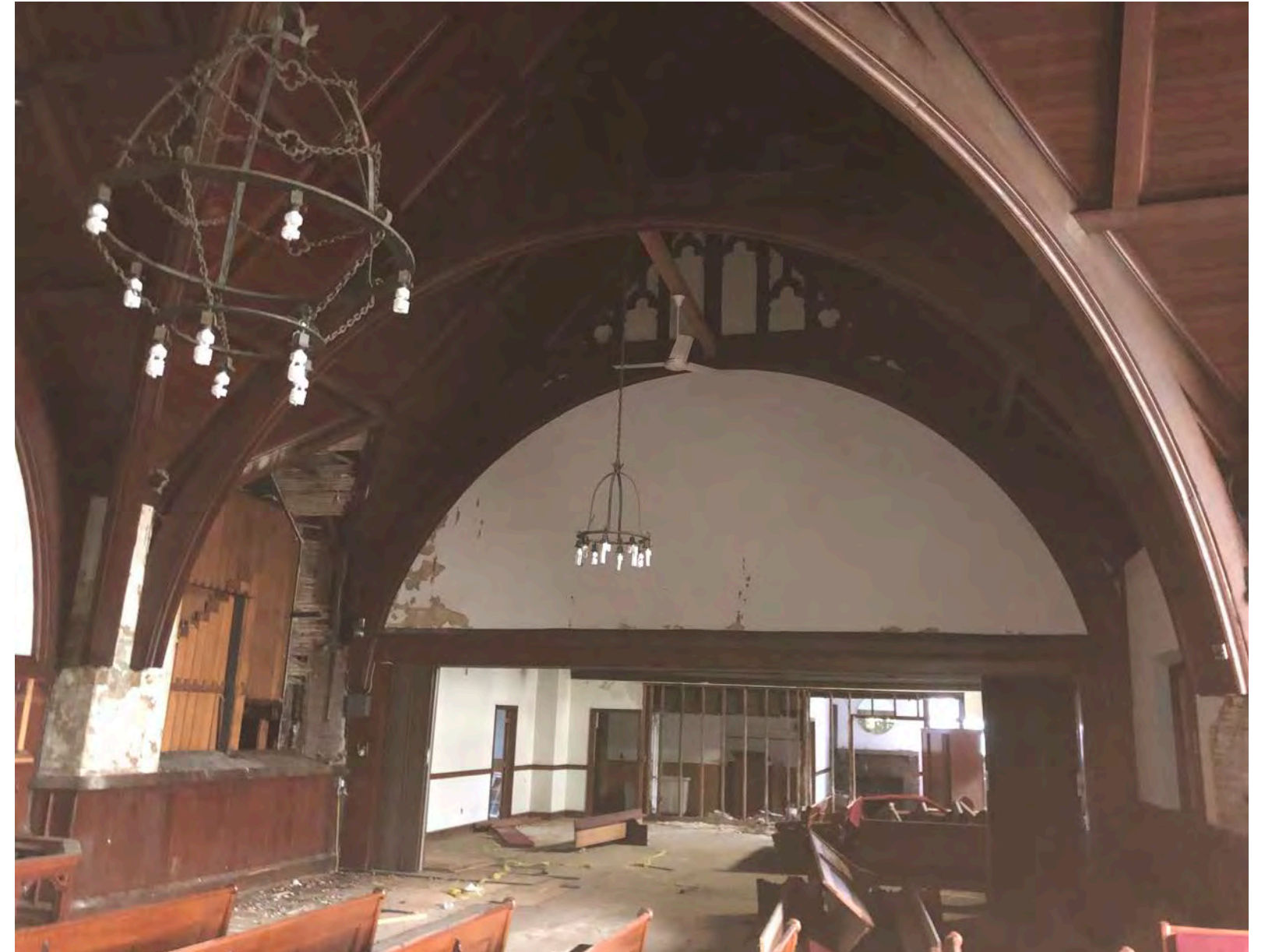
CHURCH TRANSEPT WEST
