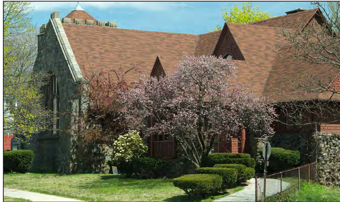
VIEW FROM HAMILTON STREET
