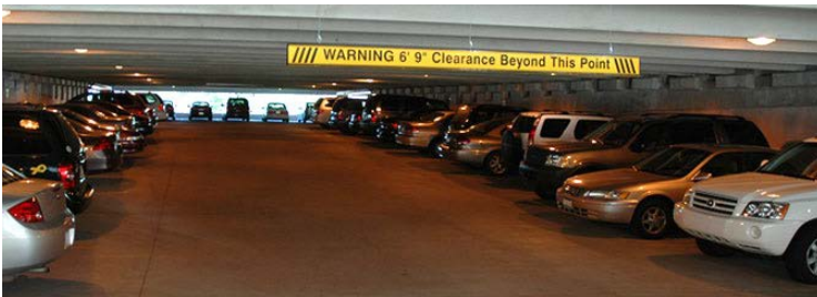
Height check at entrance of garages/bridges
