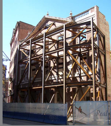
110 Westminster Street, where a historic facade faces the possibility of demolition to make way for another surface parking lot in Downcity.
