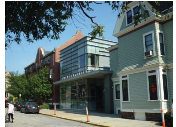
Wheeler School addition
