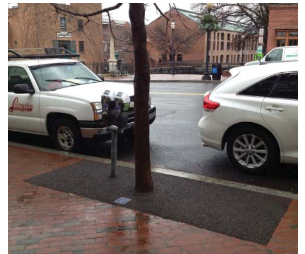
Flexi-Pave street tree pit, Washington D.C.
