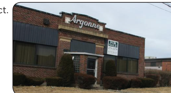
It is vital for Providence to provide opportunities for industries and industrial expansion which will employ residents of Providence, while ensuring minimal impact on adjacent residential areas.
