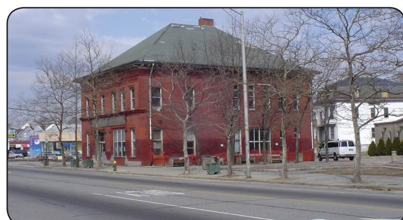
The Washington Park Branch Library was closed in 2006 due to structural and water damage issues. After renovations, the library was re-opened in March 2009.
