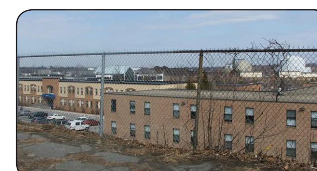
Johnson and Wales University Harborside Campus buildings.
