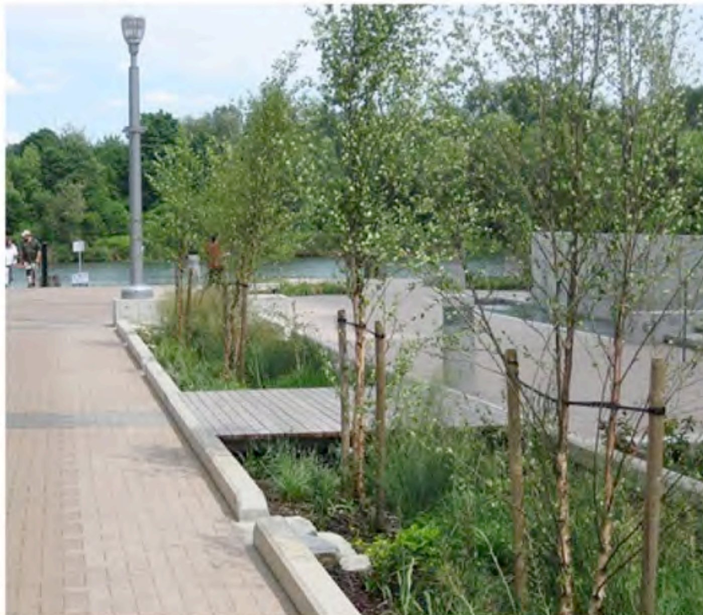
Waterfront Plaza - Portland, OR- Bioretention with Bridges and Curb Cuts
