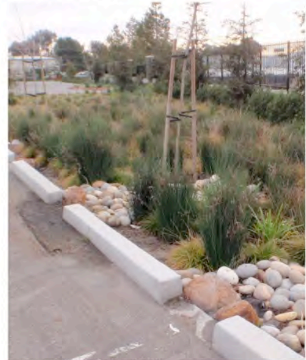
Commercial Plaza - California - Parking Perimeter Bioretention
