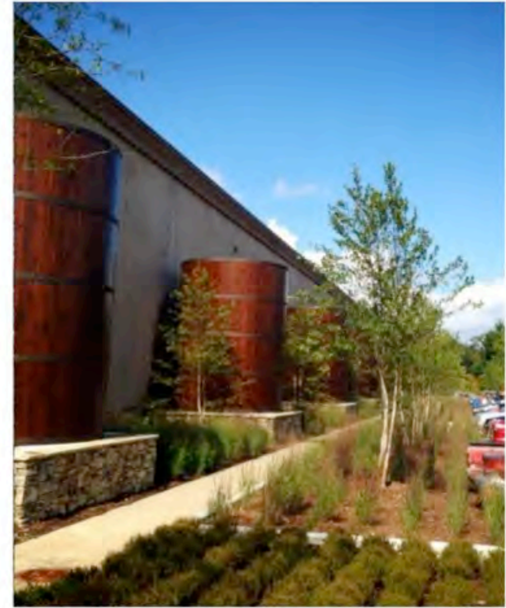
Sierra Nevada Brewery - Asheville NC - LEED Platinum facility utilizes permeable paving, captured runoff irrigation and multi-level bioretention
