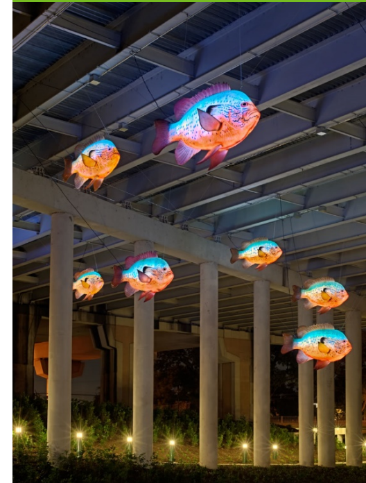
The decommissioned support platform in the river under the I-95 overpass
