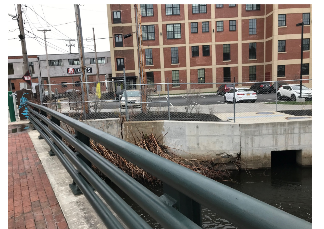
Concrete Walls Along River
