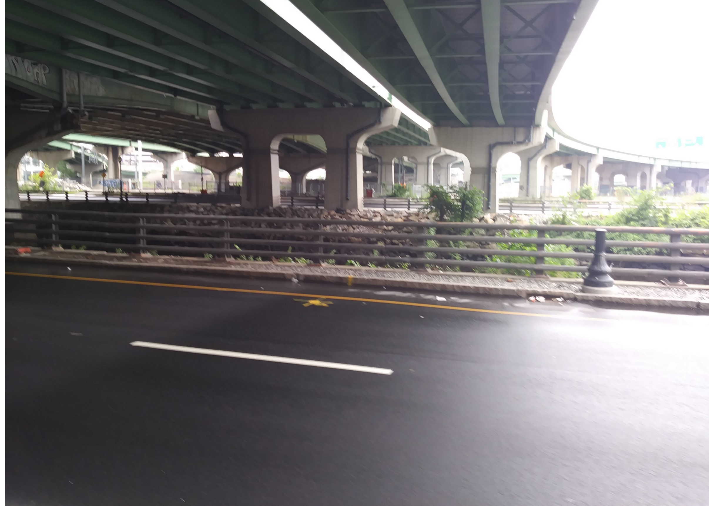
Providence Place Mall Underpass
