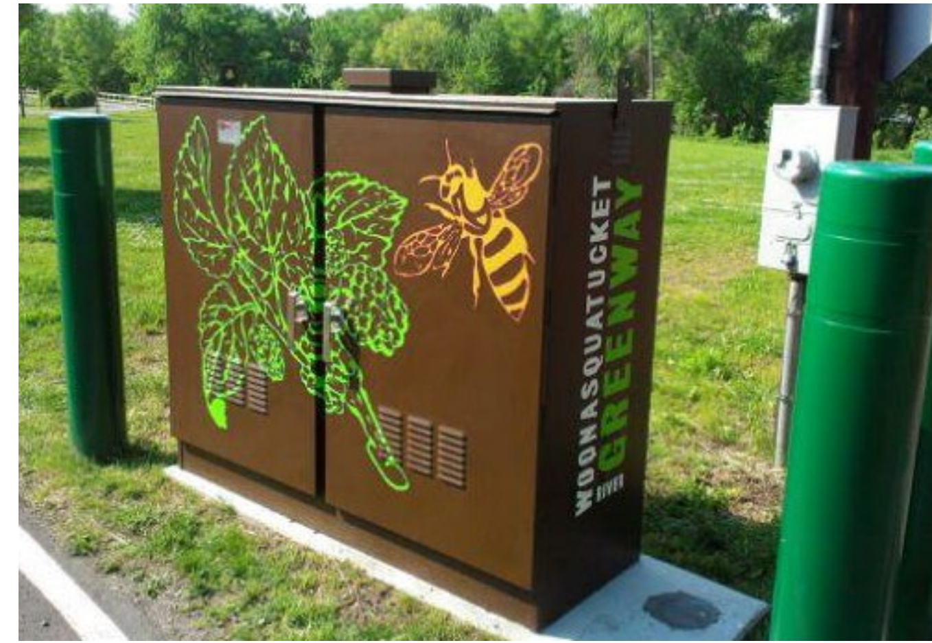
Pedestrian Bridge Sheridan Painted Electrical Boxes
