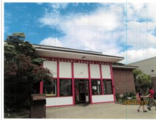
Mt. Pleasant Library Façade (After)
