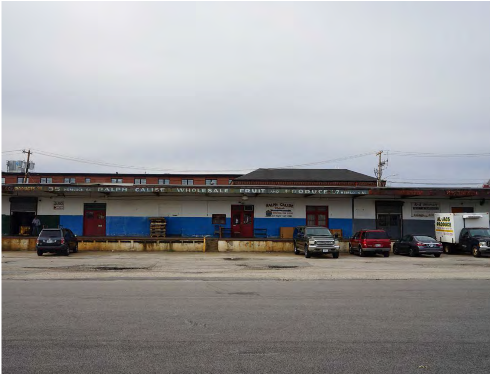
View east at fruit warehousing buildings on the Narraganset Bay Commission site.
