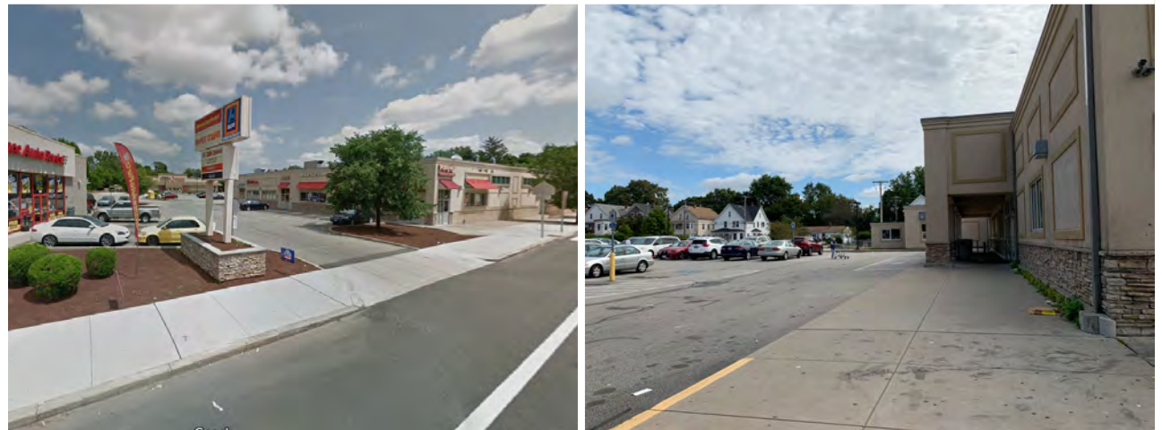
| Approaching the ALDI commercial area (Left) and the parking lot/entrance to the ALDI grocery store (Right)
