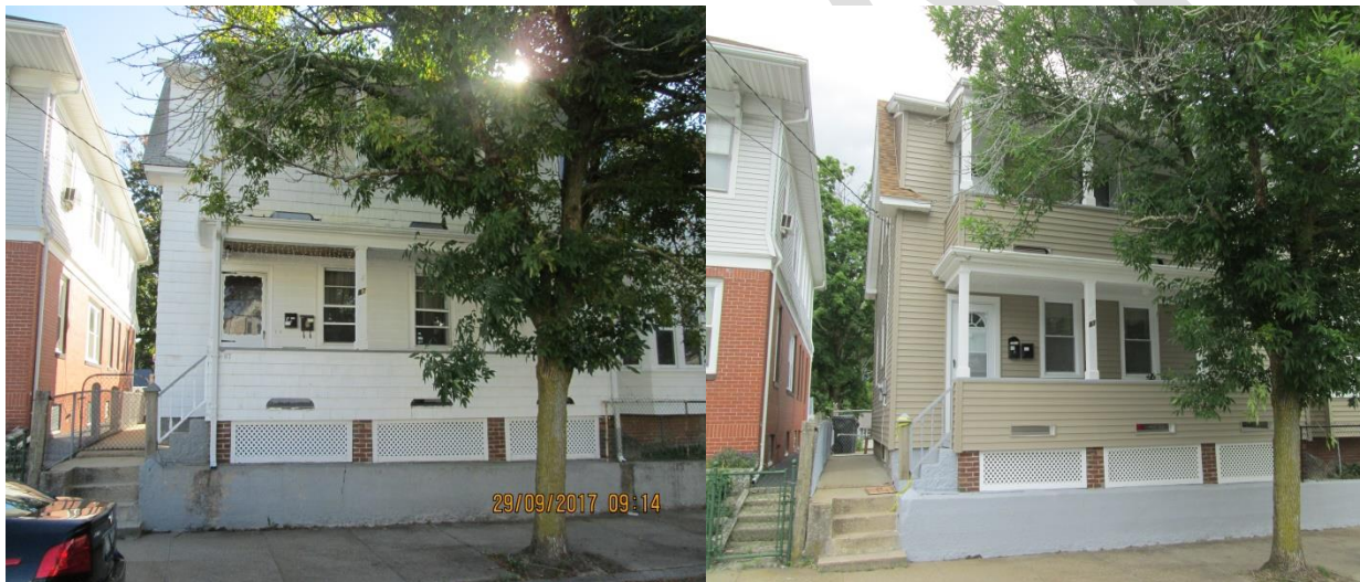
The property above received new siding, painting, and a roof replacement in 2018 through its enrollment in the CDBG Home Repair & Lead Safe Providence Programs.
