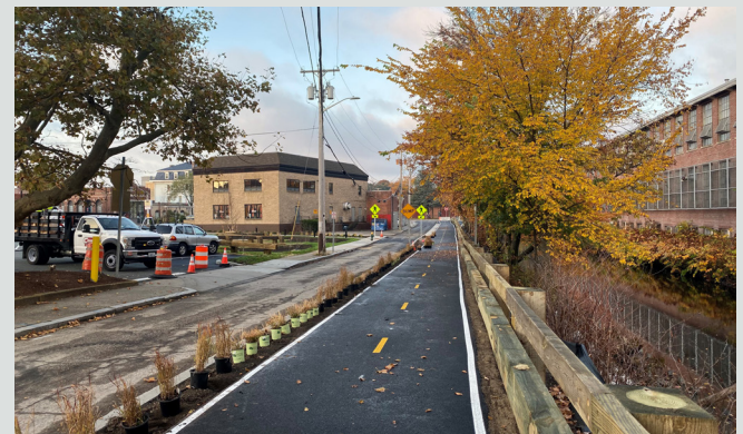
After: Substantial completion in October 2019
