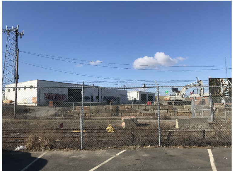
Image of existing conditions
