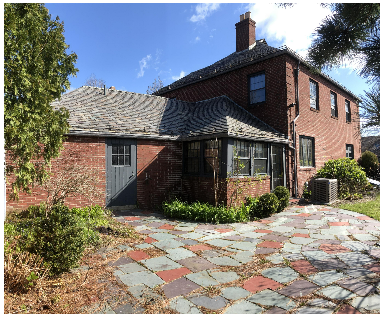
SOUTH (REAR) FACADE - VIEW FROM REAR YARD AT SOUTHWEST CORNER (BREAKFAST ROOM AT CENTER OF PHOTO TO BE DEMOLISHED TO ACCOMMODATE CONSERVATORY ADDITION)
