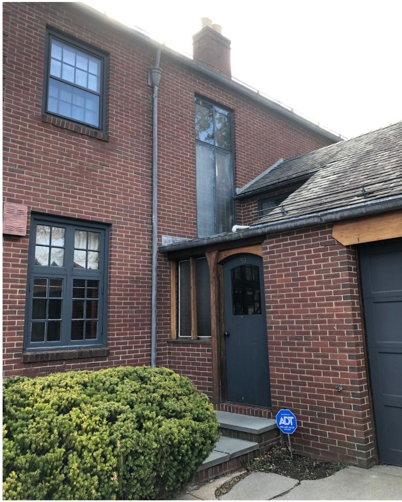
NON-ORIGINAL VESTIBULE AT SECONDARY ENTRY (TO BE REMOVED): VIEW FROM DRIVEWAY
