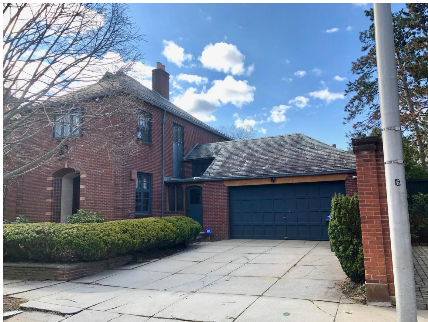
NORTH (FRONT) FACADE - VIEW FROM STIMSON AVENUE AT NORTHWEST CORNER OF PROPERTY (VARNISHED GARAGE DOOR HEADER TRIMBOARD AND NON-ORIGINAL SECONDARY ENTRY VESTIBULE (TO BE REMOVED) VISIBLE AT RIGHT SIDE OF PHOTO)
