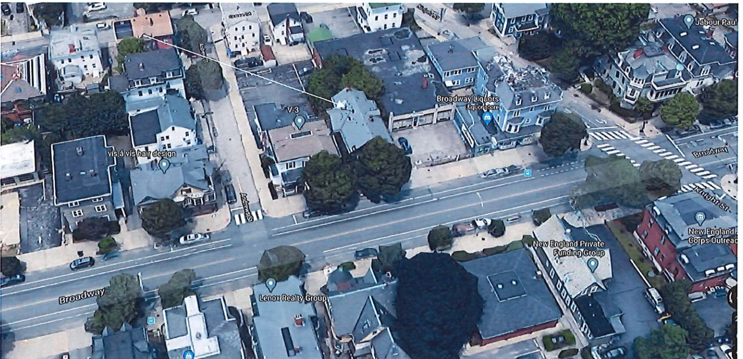
Arrow indicates project location, looking north.
