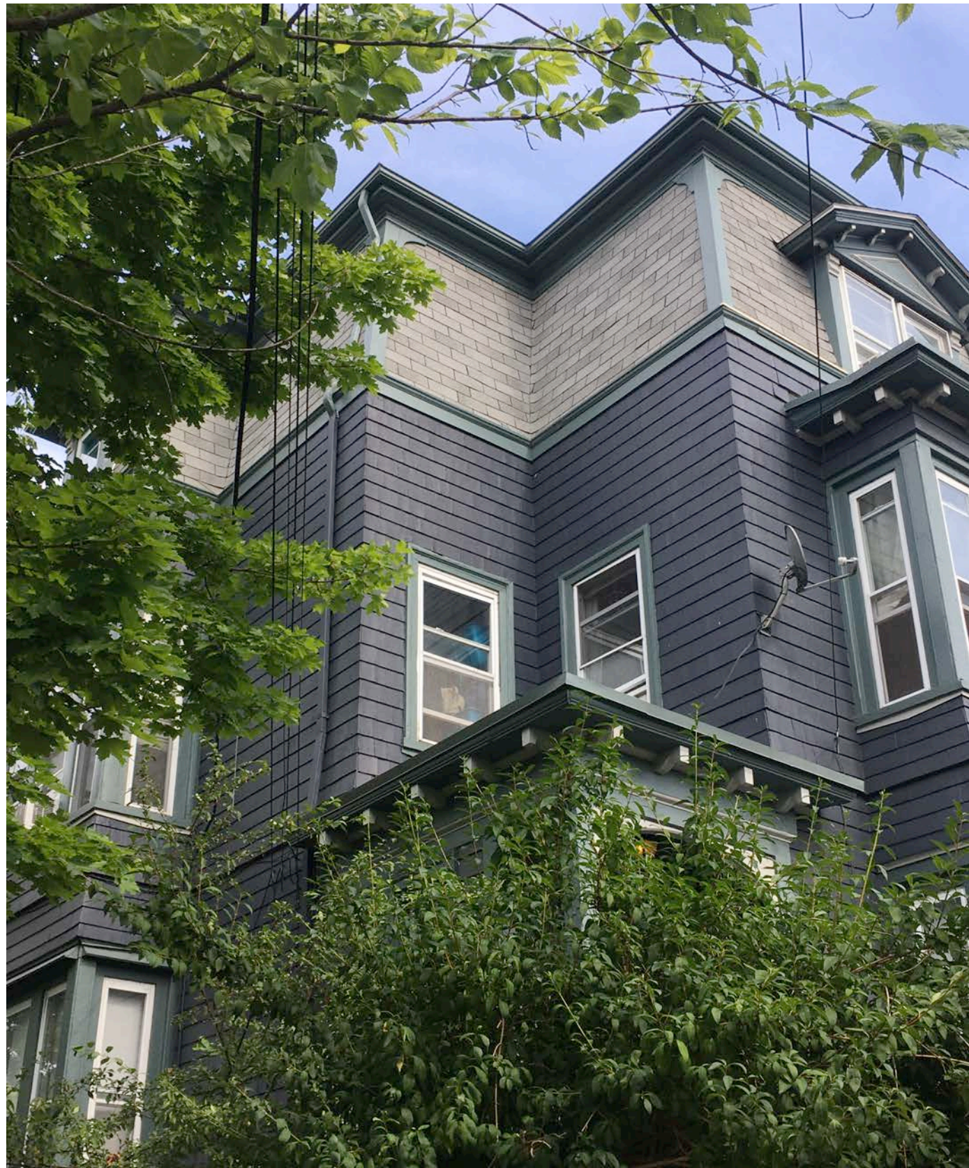
① EXISTING DETAIL PHOTO (NORTHWEST) Roof Area
