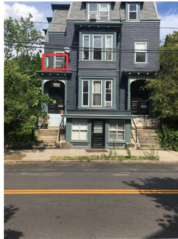
2 View from West showing area of work 20-22 Messer Street
