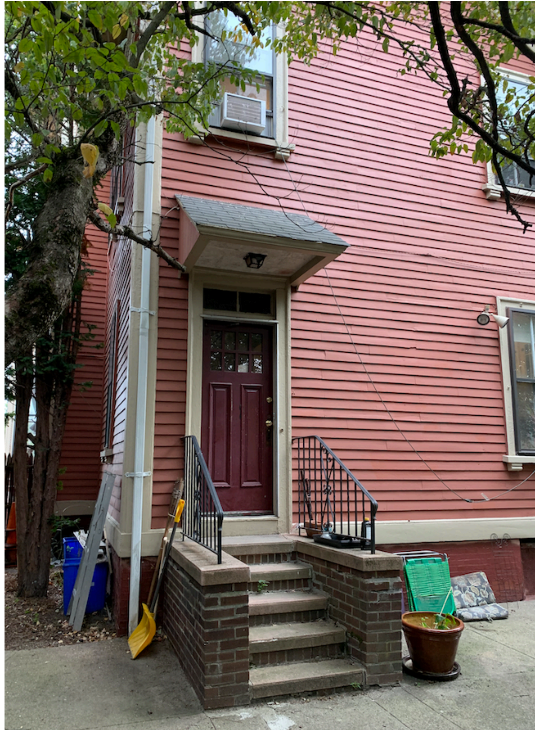
Rotate Existing Masonry Stoop- existing awning to remain, masonry stoop to be removed and reconstructed 90 degrees relative to existing condition as shown
