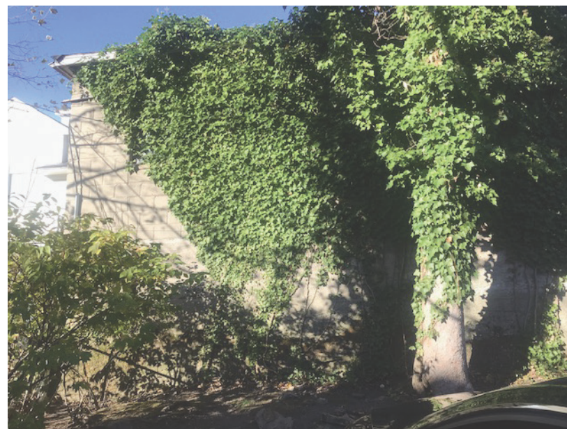
Existing CMU / Concrete Wall at Garage South (Back) Elevation
