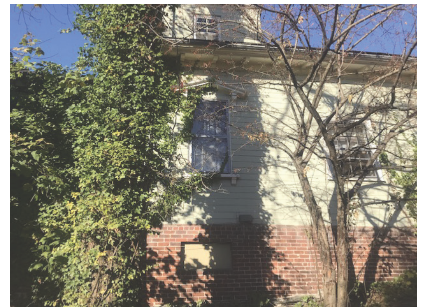
Existing Brick / Wood Siding Wall at Cottage South (Back) Elevation
