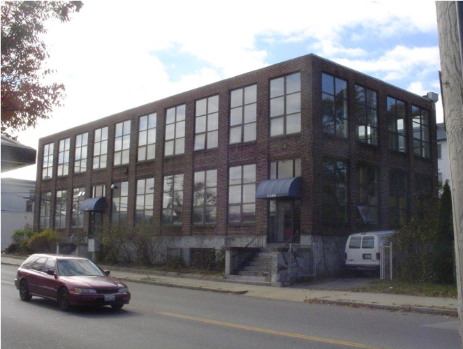
View of the building from Eddy Street
