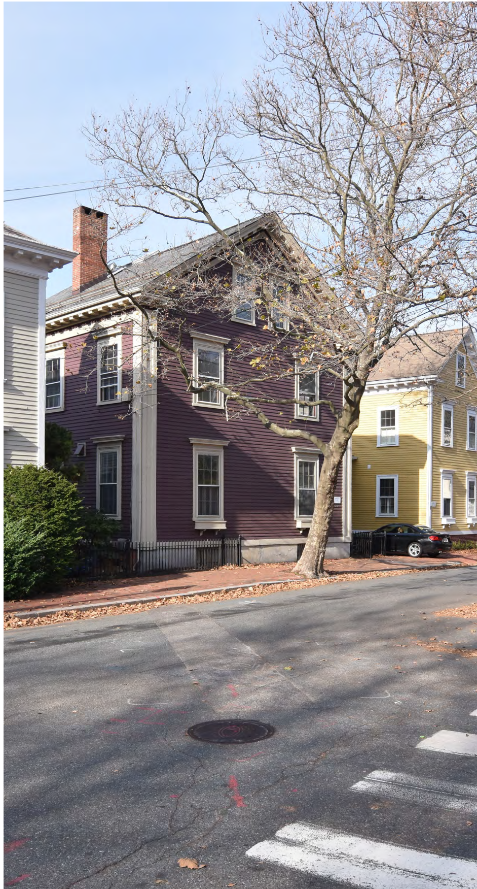
EXISTING CONDITION - VIEW FROM BENEFIT STREET
