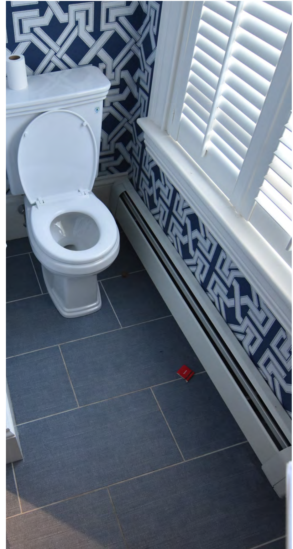
EXISTING CONDITION SECOND FLOOR BATH
