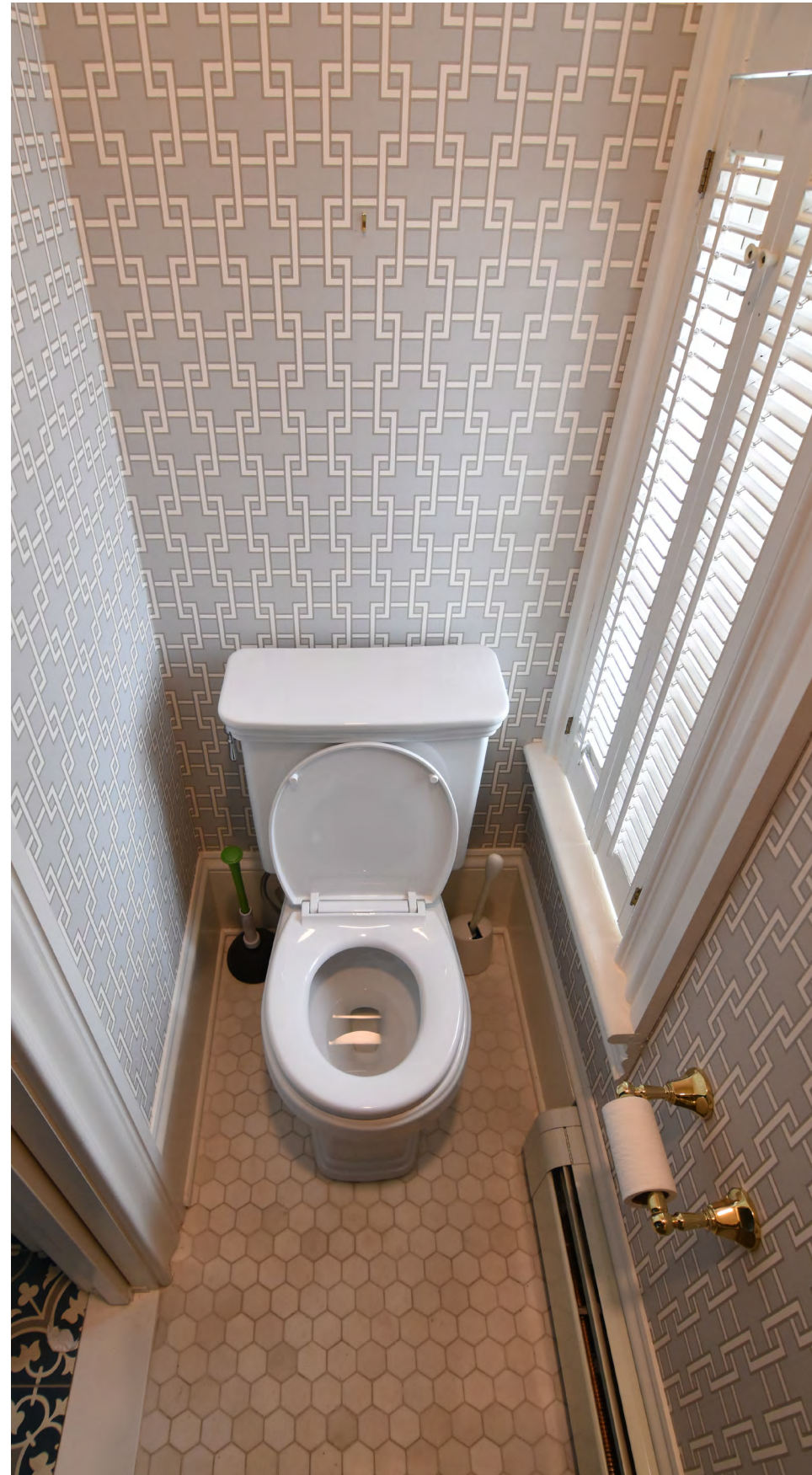
EXISTING CONDITION FIRST FLOOR WATER CLOSET WINDOW
