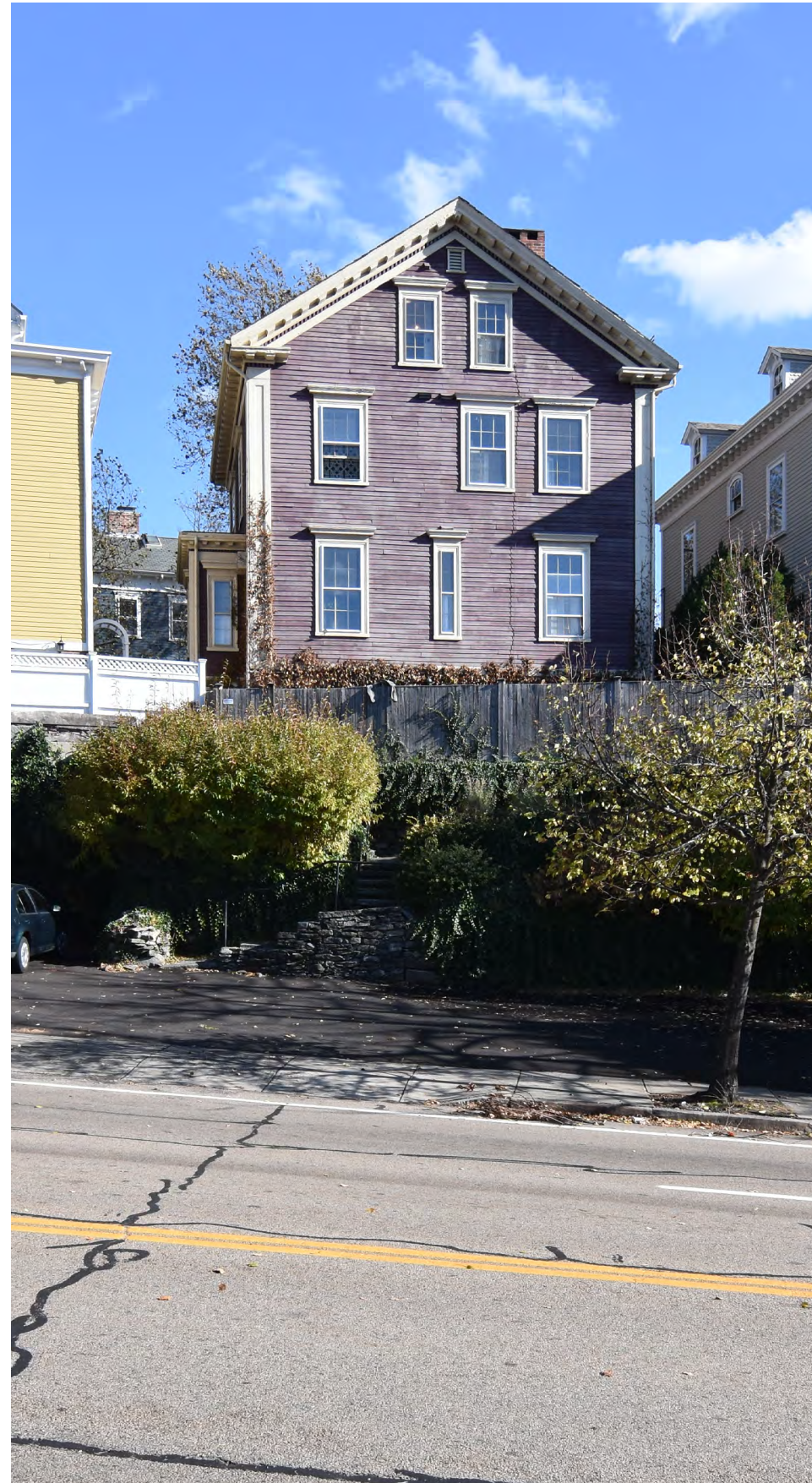
EXISTING CONDITION - REAR ELEVATION
