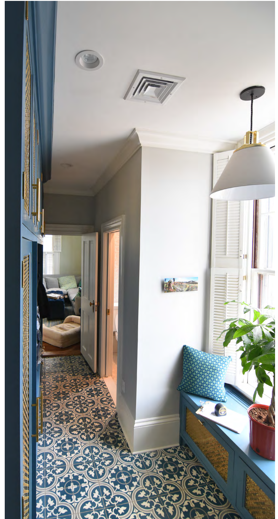
EXISTING CONDITION FIRST FLOOR MUDROOM WINDOW
