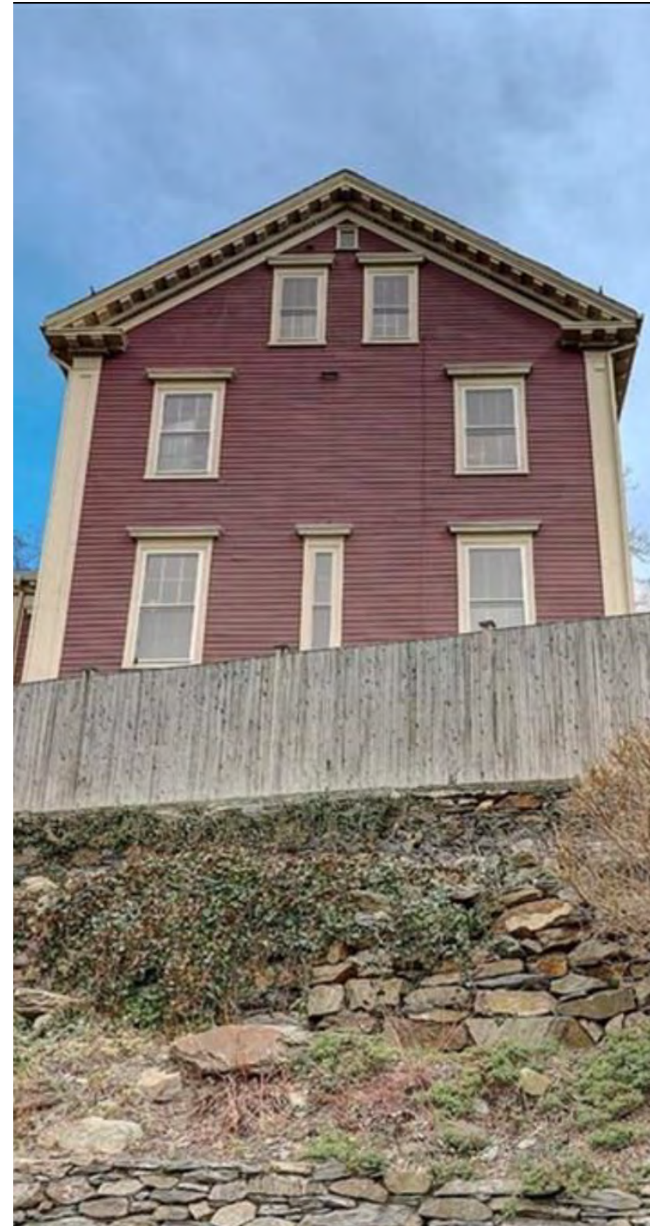
RECENT CONDITION OF REAR ELEVATION
