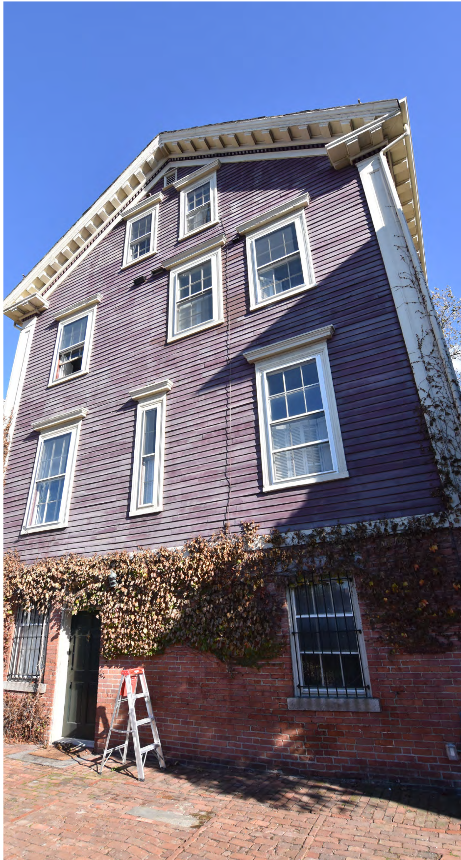
EXISTING CONDITION - REAR ELEVATION
