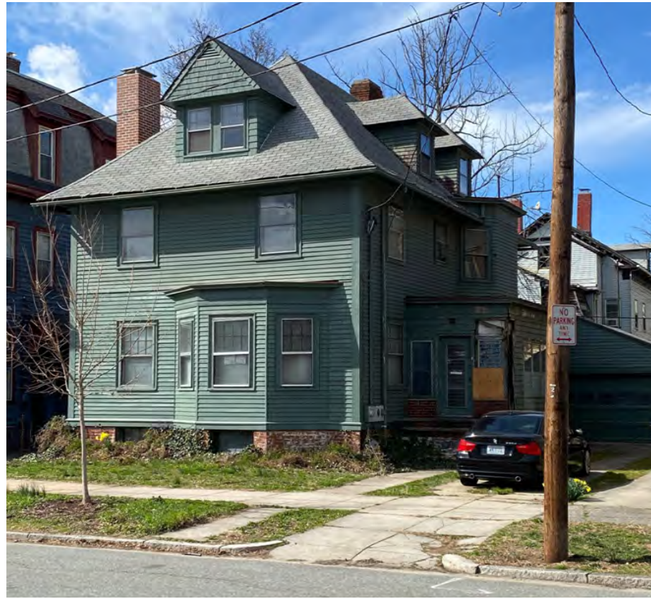
27 HOLLYWOOD ROAD - VIEW FROM RIGHT
