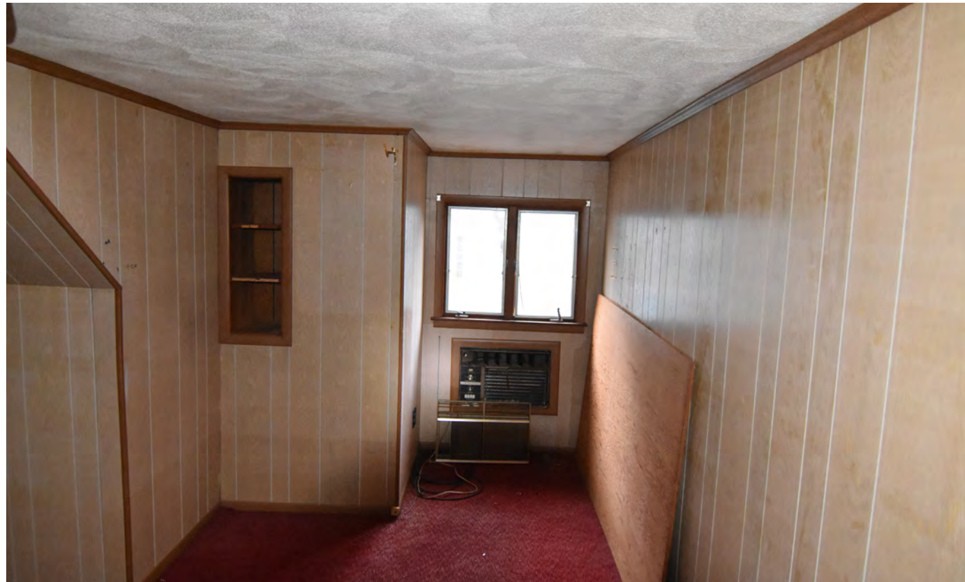
EXISTING CONDITION SECOND FLOOR
