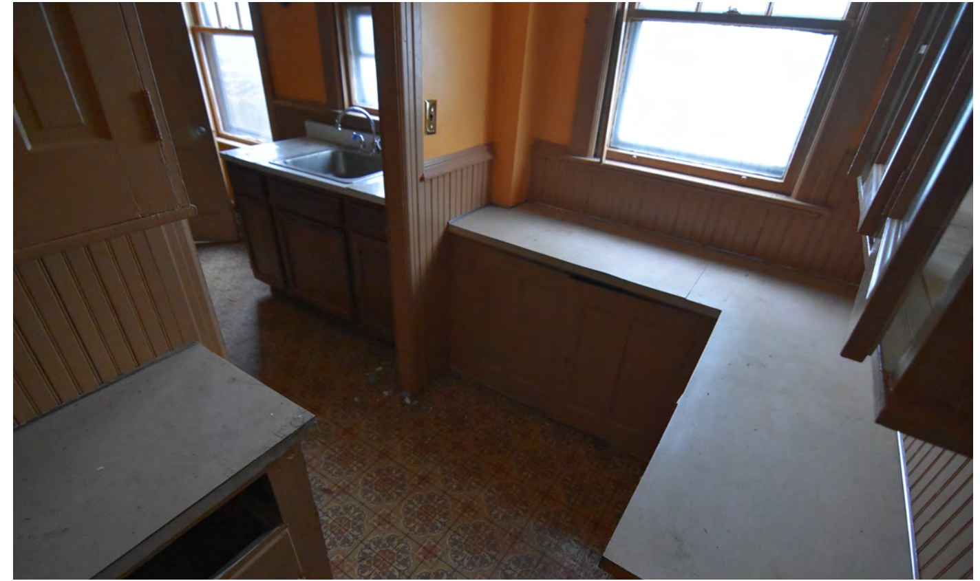
EXISTING CONDITION FIRST FLOOR PANTRY
