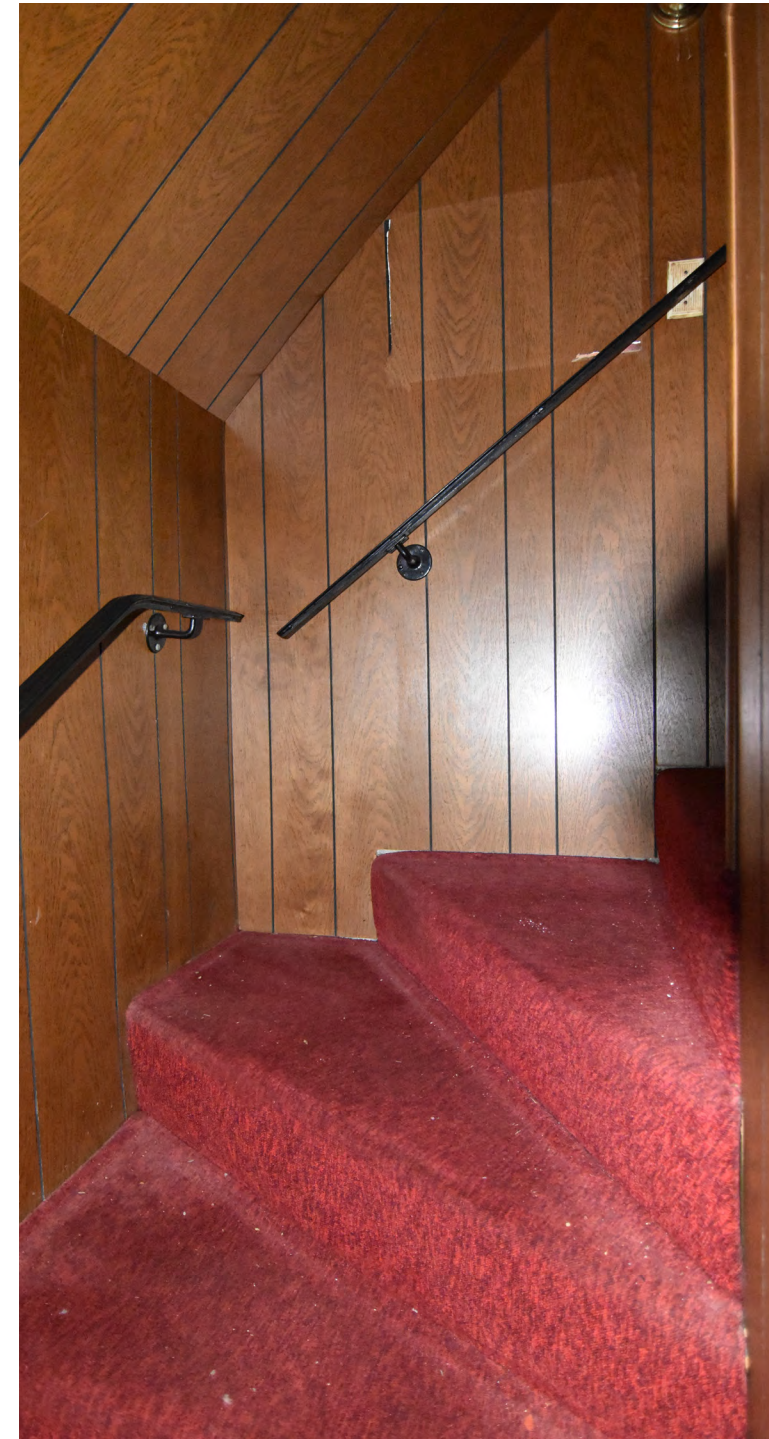
EXISTING CONDITION STAIR TO SECOND FLOOR
