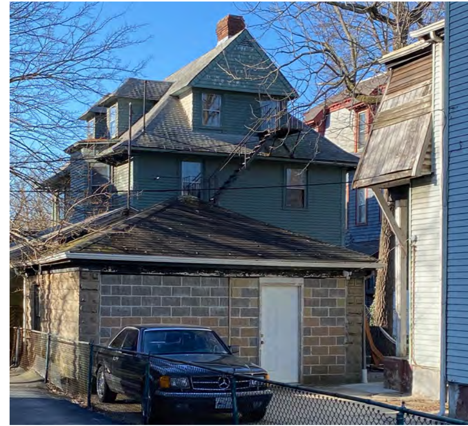
27 HOLLYWOOD ROAD - REAR SIDE VIEW
