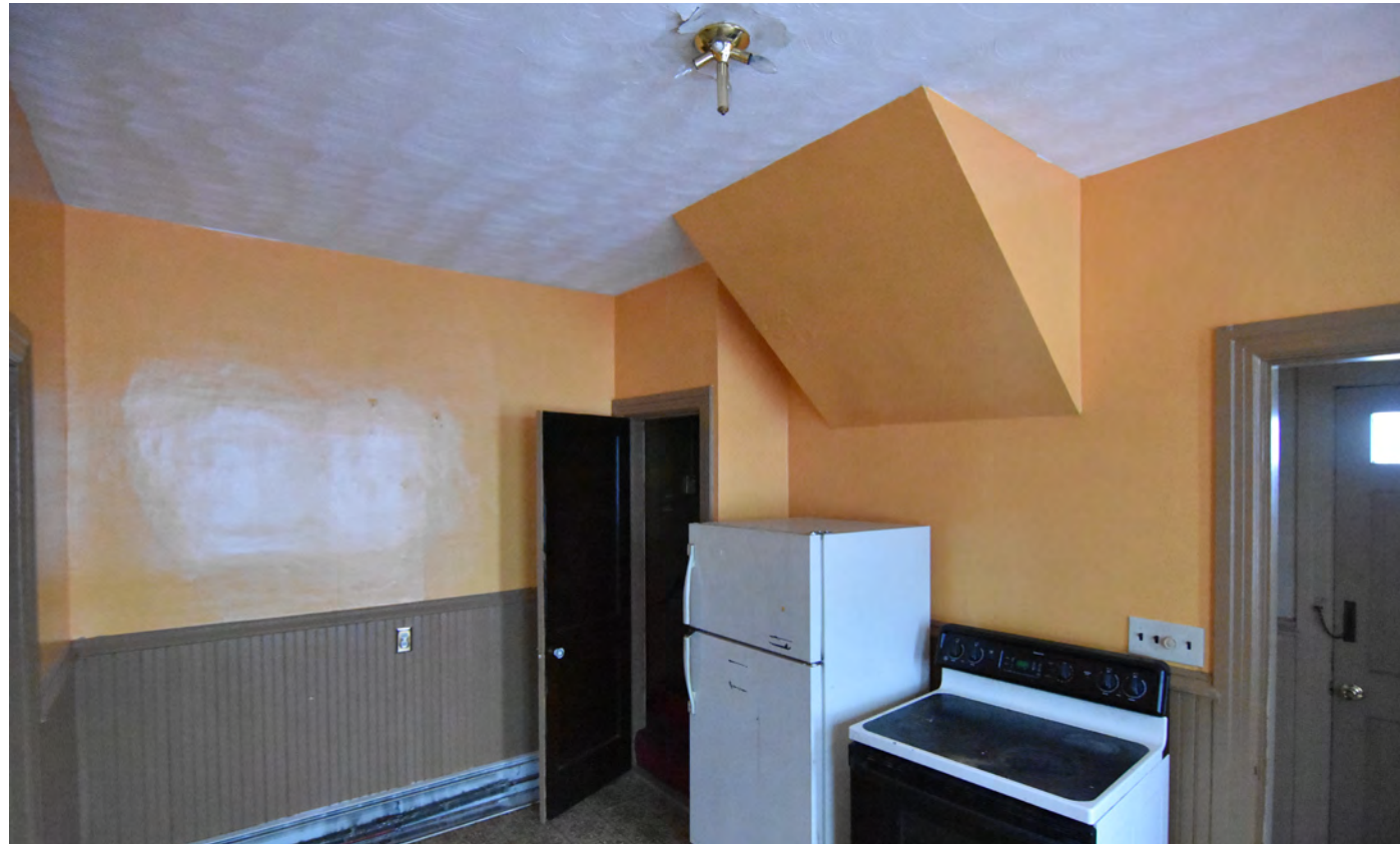
EXISTING CONDITION FIRST FLOOR KITCHEN
