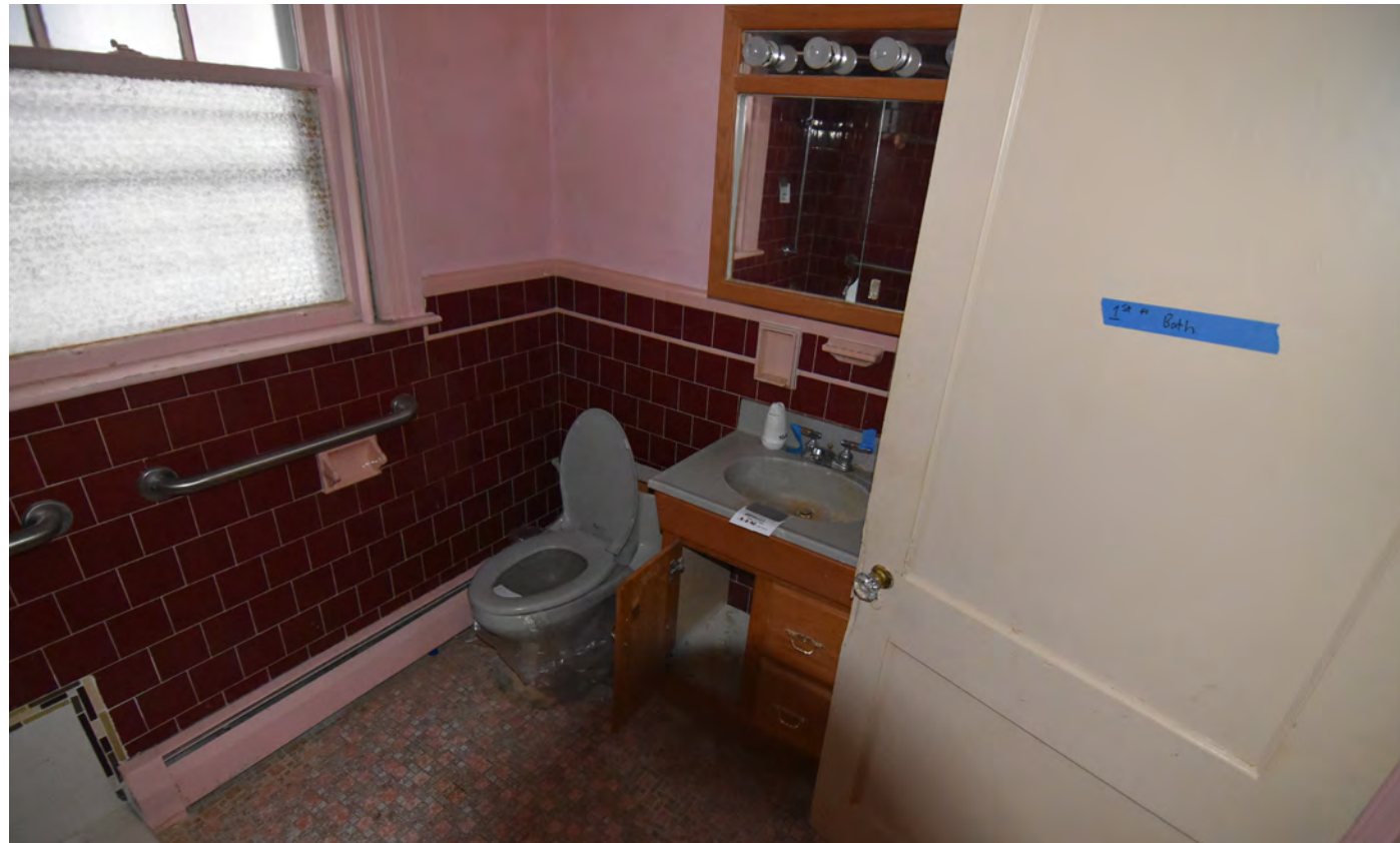
EXISTING CONDITION FIRST FLOOR BATH
