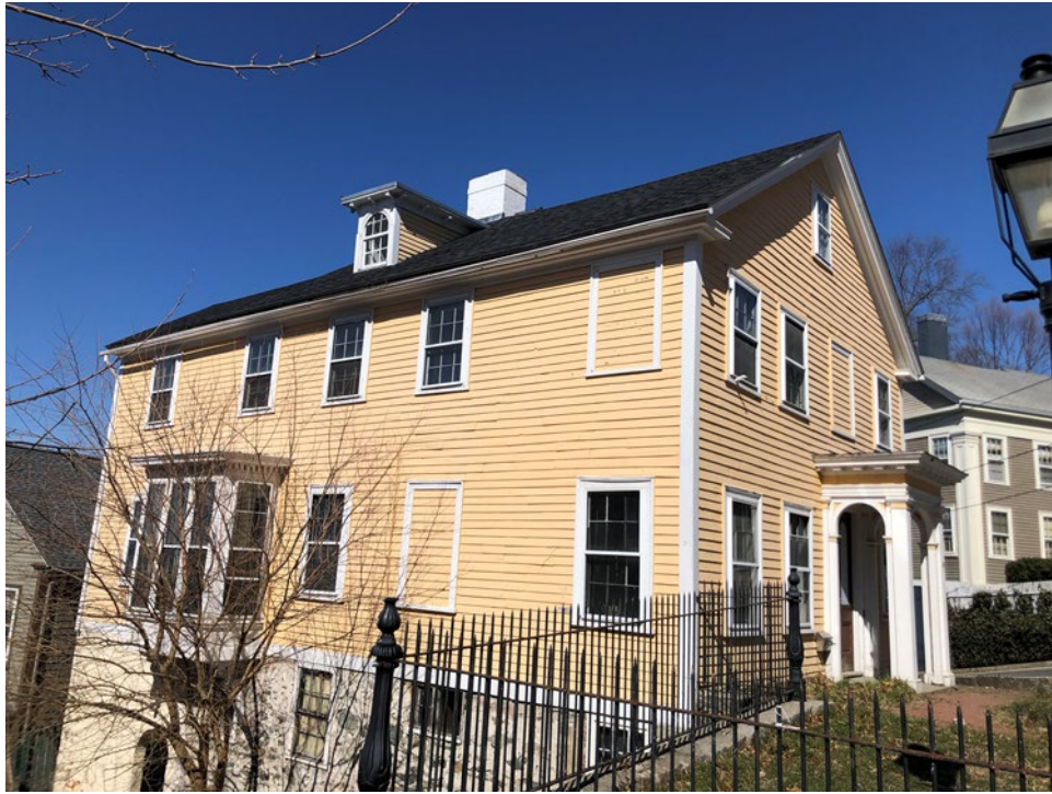
6 - View from Meeting Street stair
