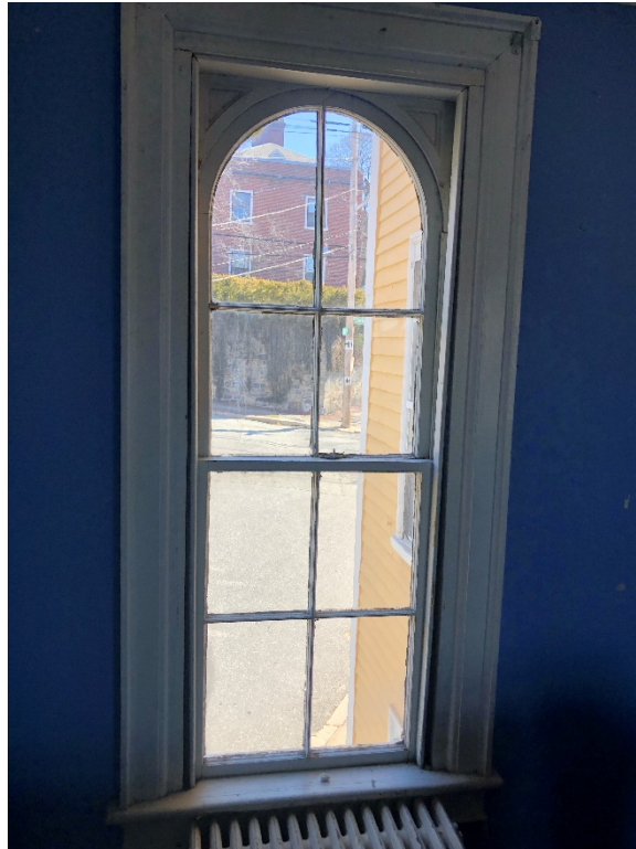
11 - Arch sash in square frame - Unit "K"
