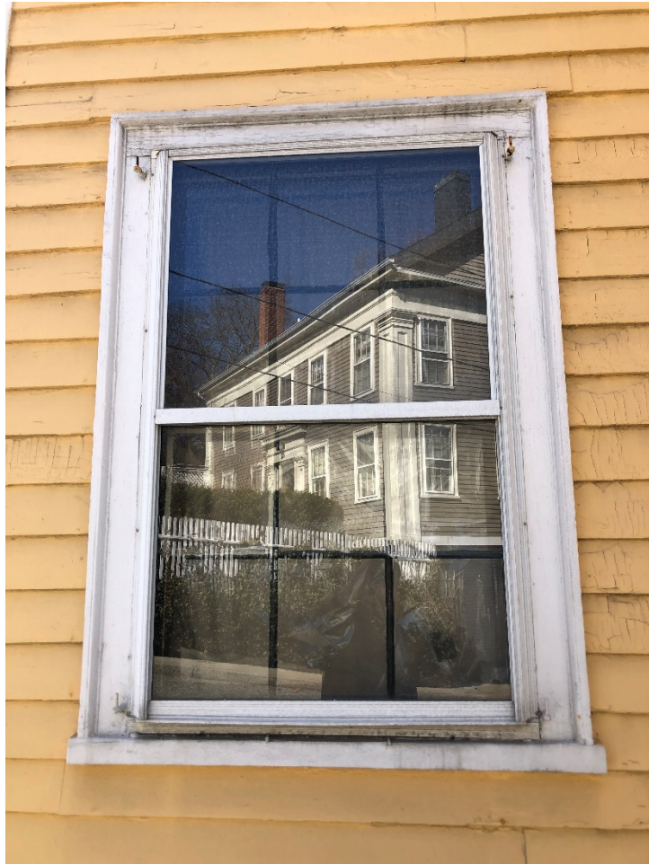
8 - Typical exterior view
