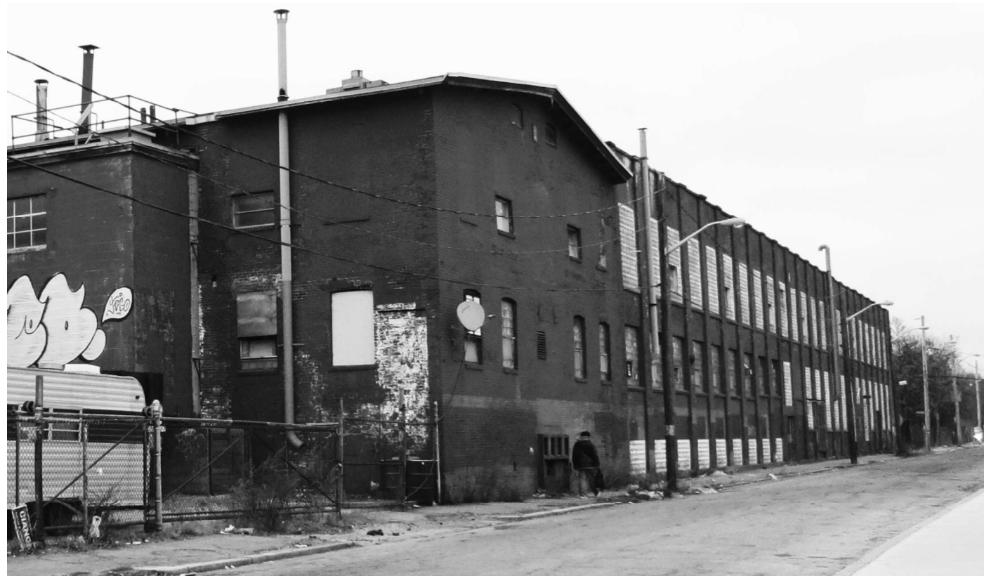
2 EXISTING PHOTOGRAPH NTS
