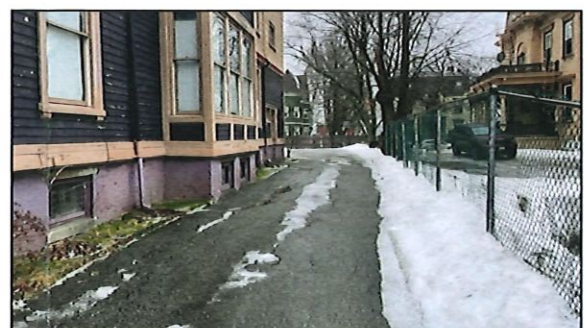
View along driveway towards Mawney St
