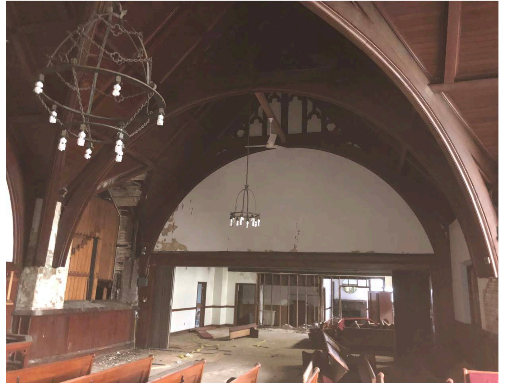
CHURCH TRANSEPT WEST
