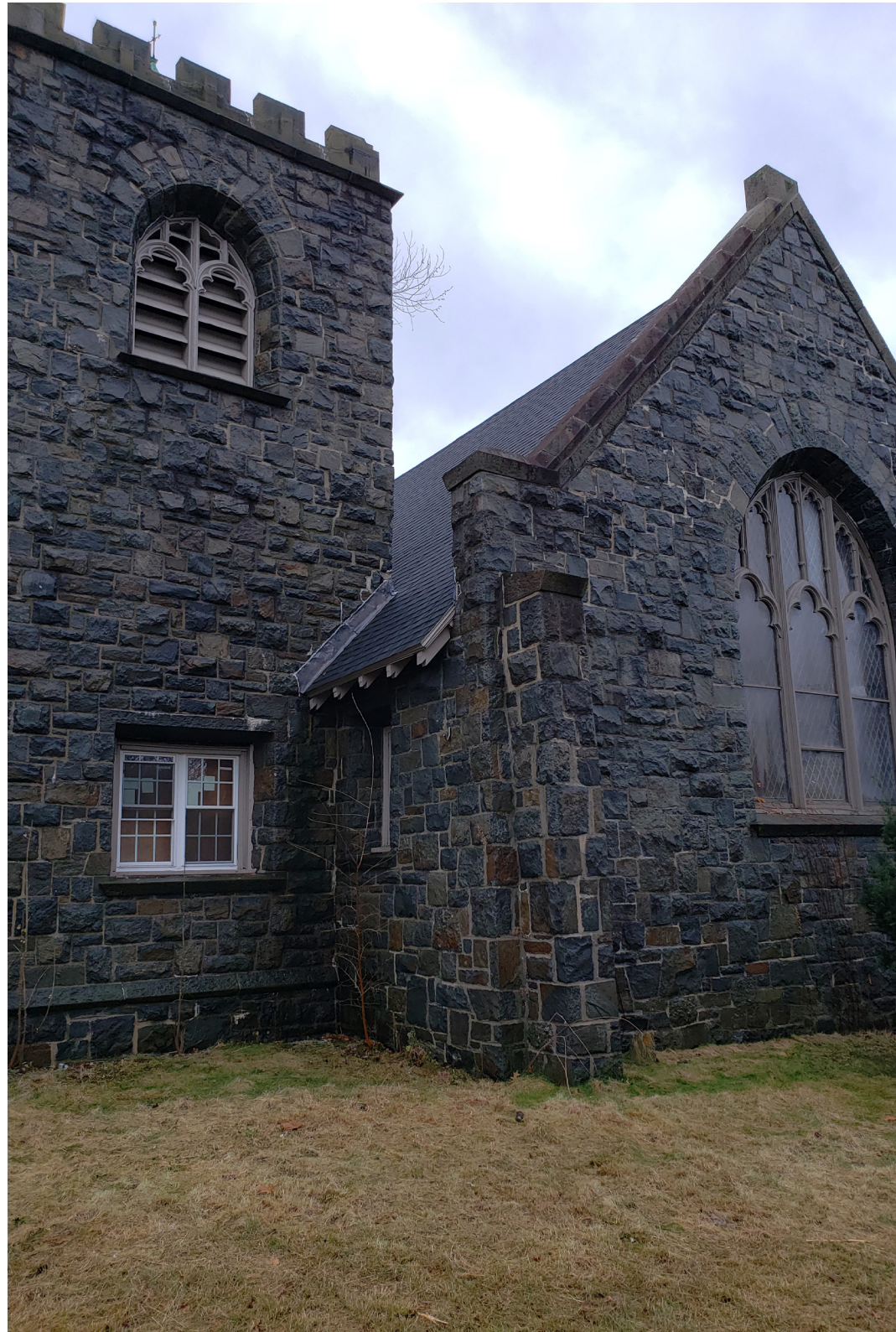
VIEW OF TOWER
