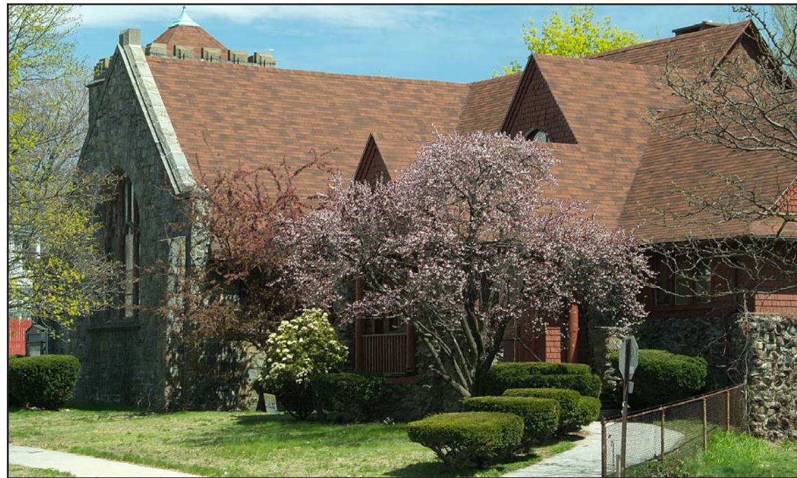
VIEW FROM HAMILTON STREET
