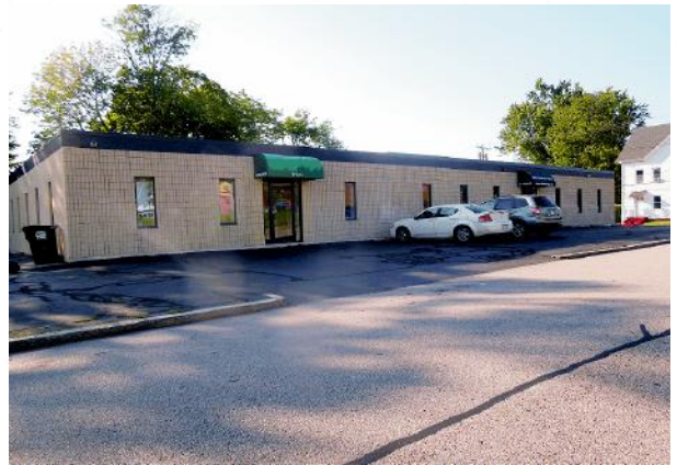
VIEW OF COMMERCIAL BUILDING AT 48 NASHUA STREET, CORNER OF FROST STREET
