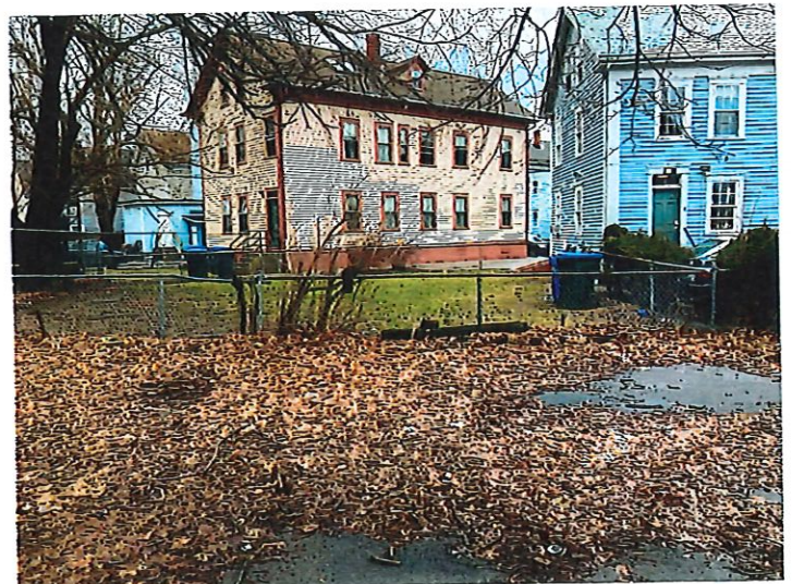
Facing North of Gilmore Street Property.
