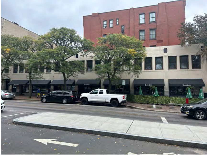
Building Front View
