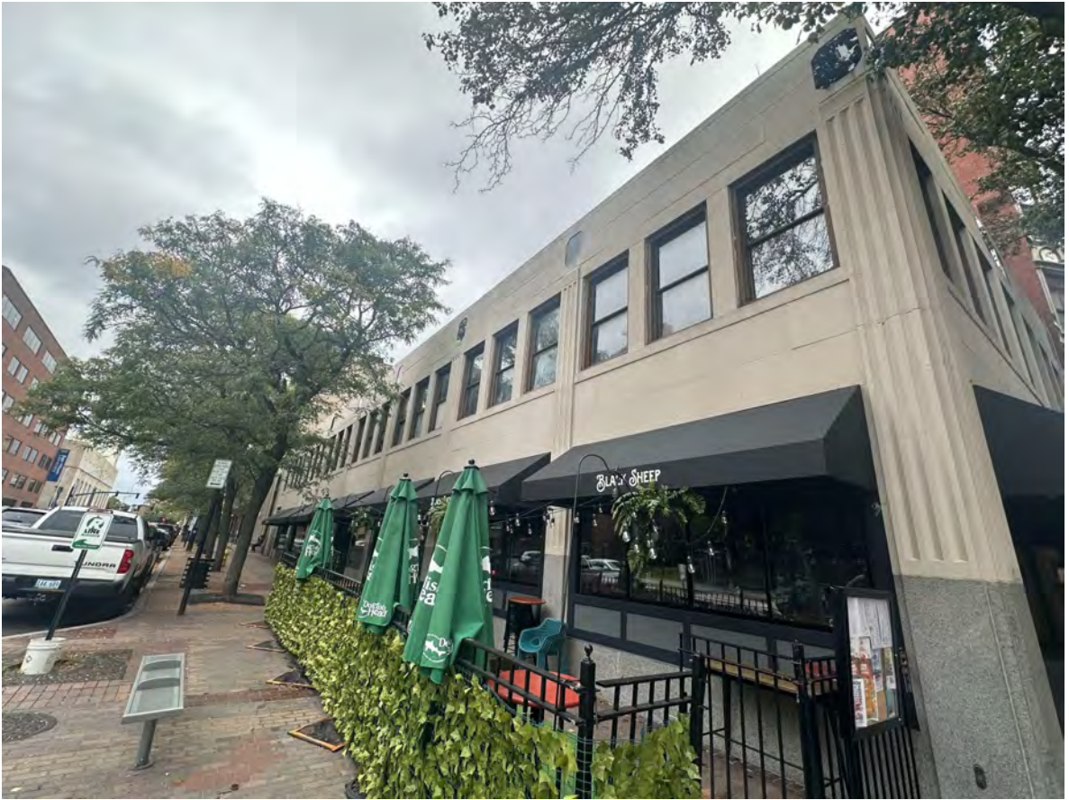
Right Side View of Building Front
