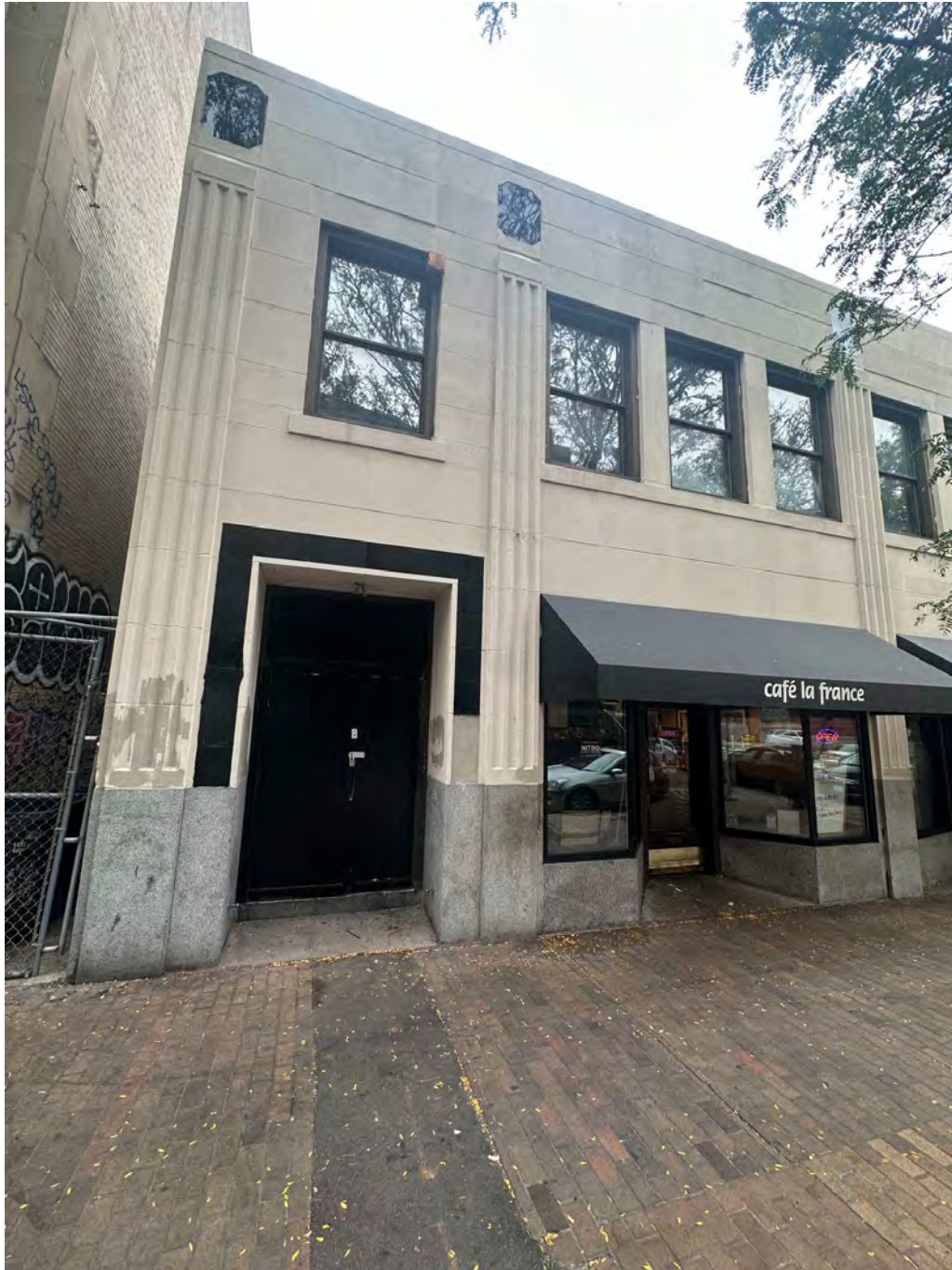
Entrance to the 2nd floor Building Front
