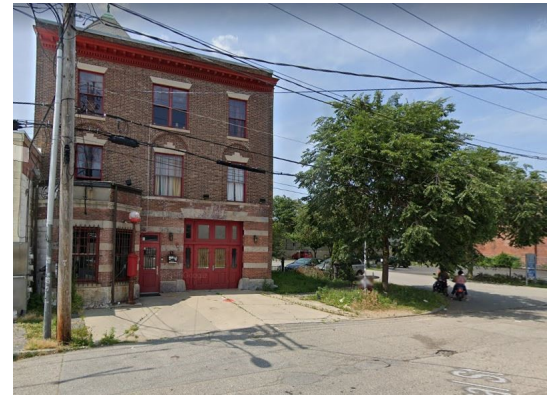
View from Central Street
