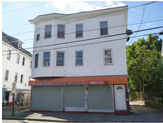
View from Plainfield Street
