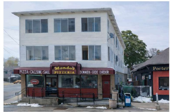
A view of the building from Admiral Street
