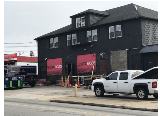
View from Valley Street
