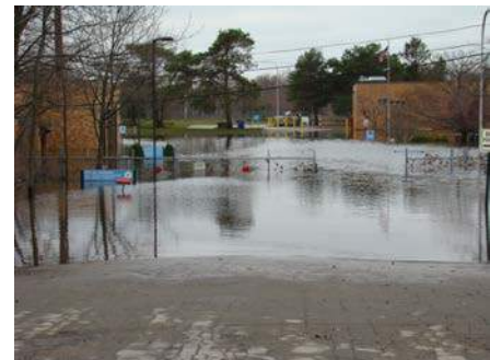
Warwick Wastewater Treatment Plant under water. Photo courtesy: City of Warwick DPW.
