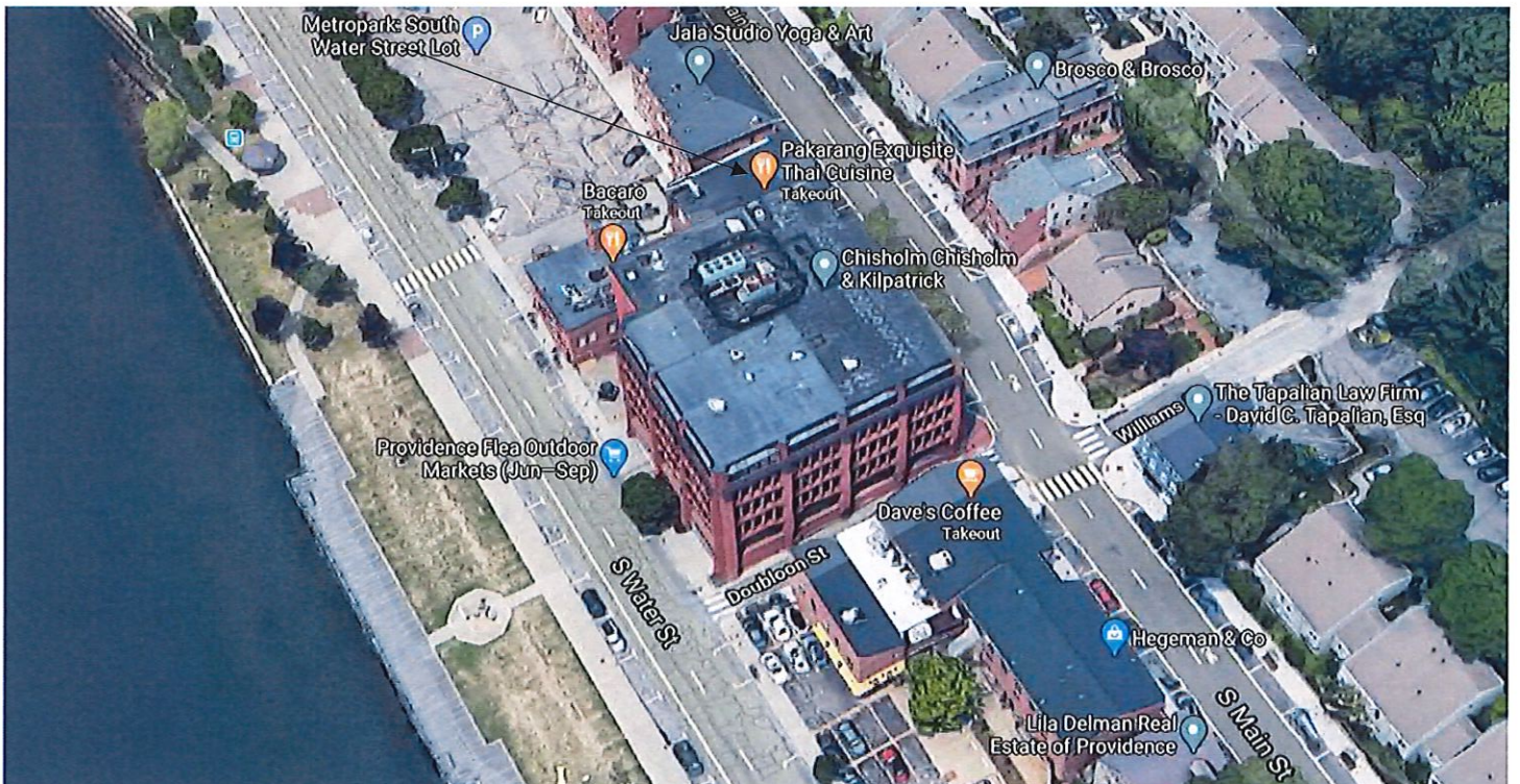
Arrow indicates project location, looking north.
