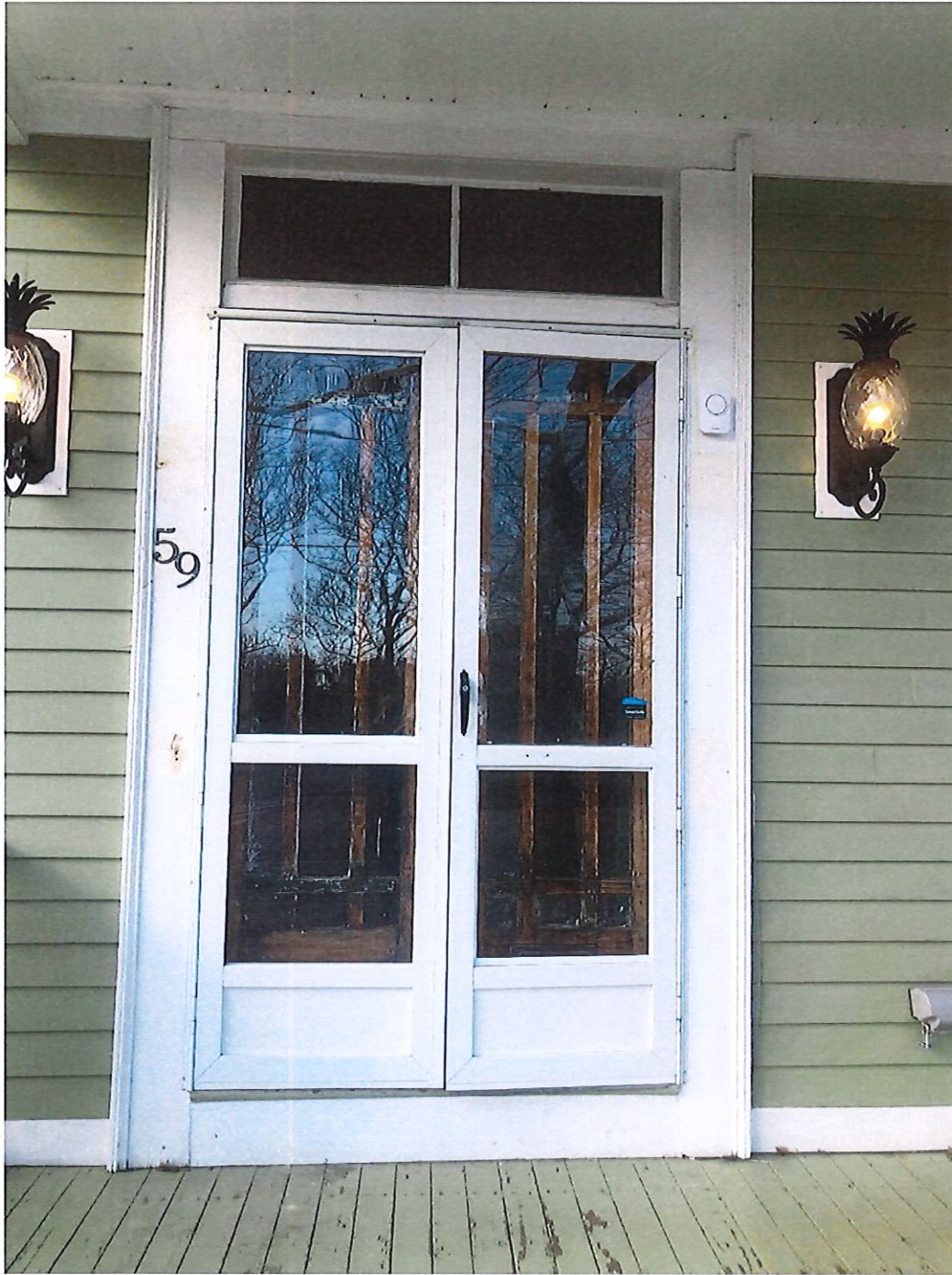
6 - Entry door - no work
