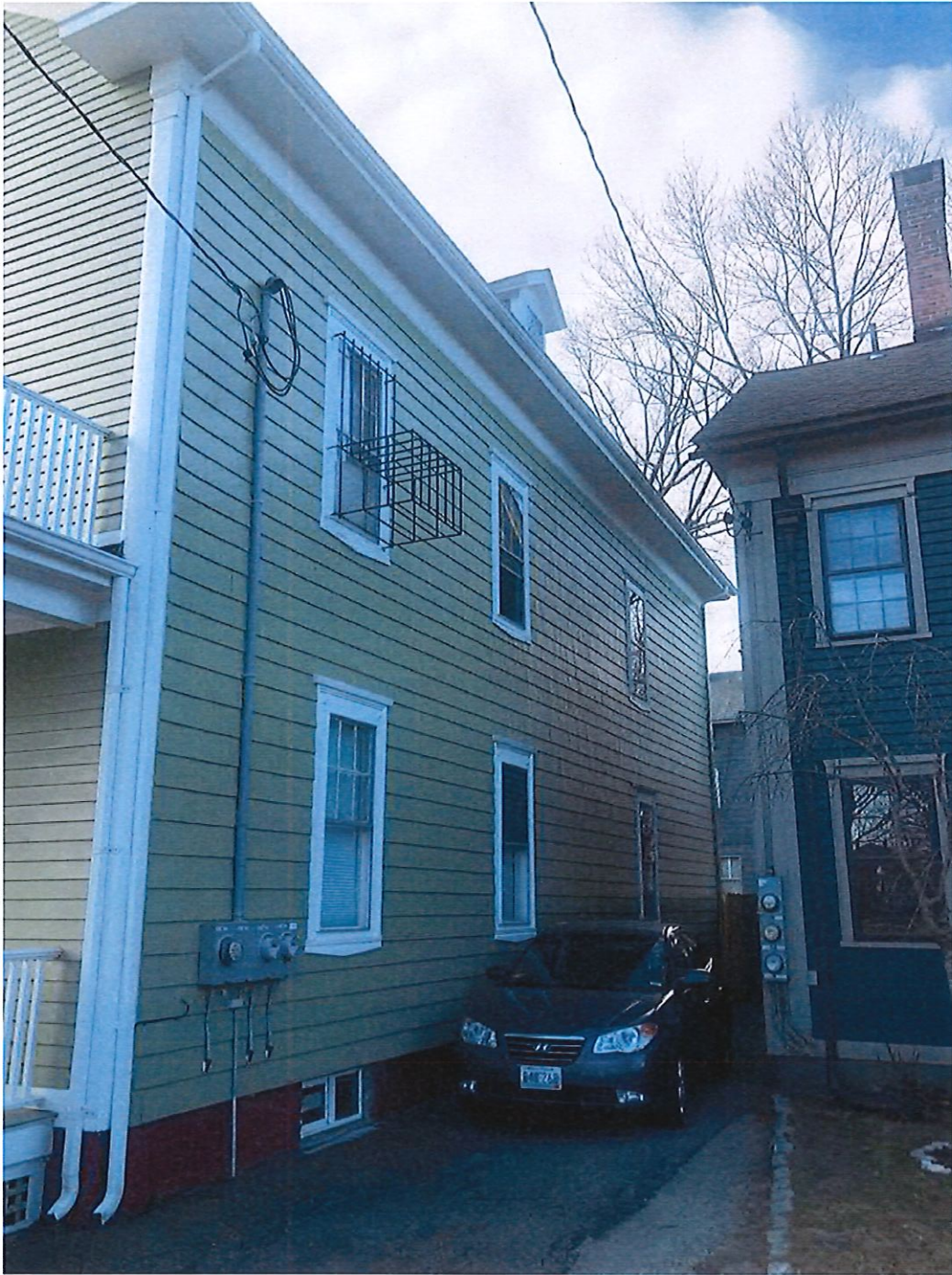
4- Side of building
