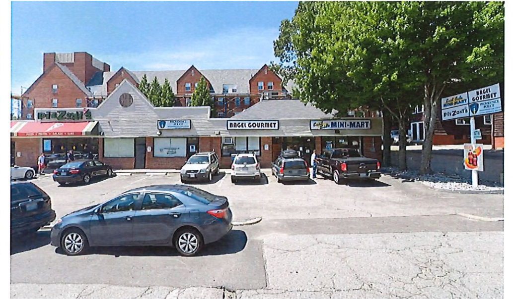
VIEW LOOKING WEST ON BROOK STREET BETWEEN POWER STREET AND CHARLESFIELD STREET
