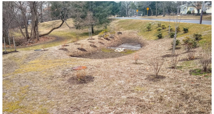
Infiltration basins use the natural filtration properties of soil to treat and infiltrate stormwater. Photos courtesy of the Stormwater Innovation Center
