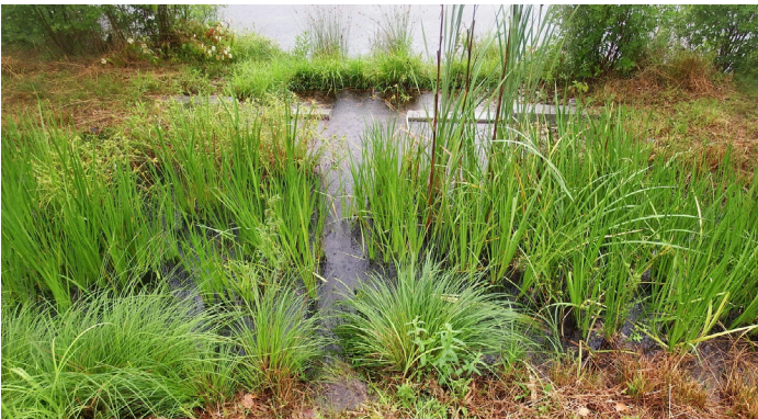
Rain gardens are an example of bioretention, they work by allowing stormwater to pool on the surface and slowly infiltrate into the ground. These photos show two rain gardens located in Roger Williams Park. Photos courtesy of the Stormwater Innovation Center
