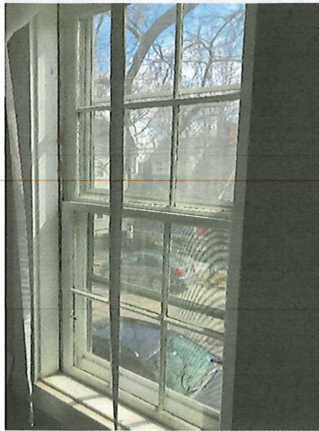
5 - 6/6 facing John Street
