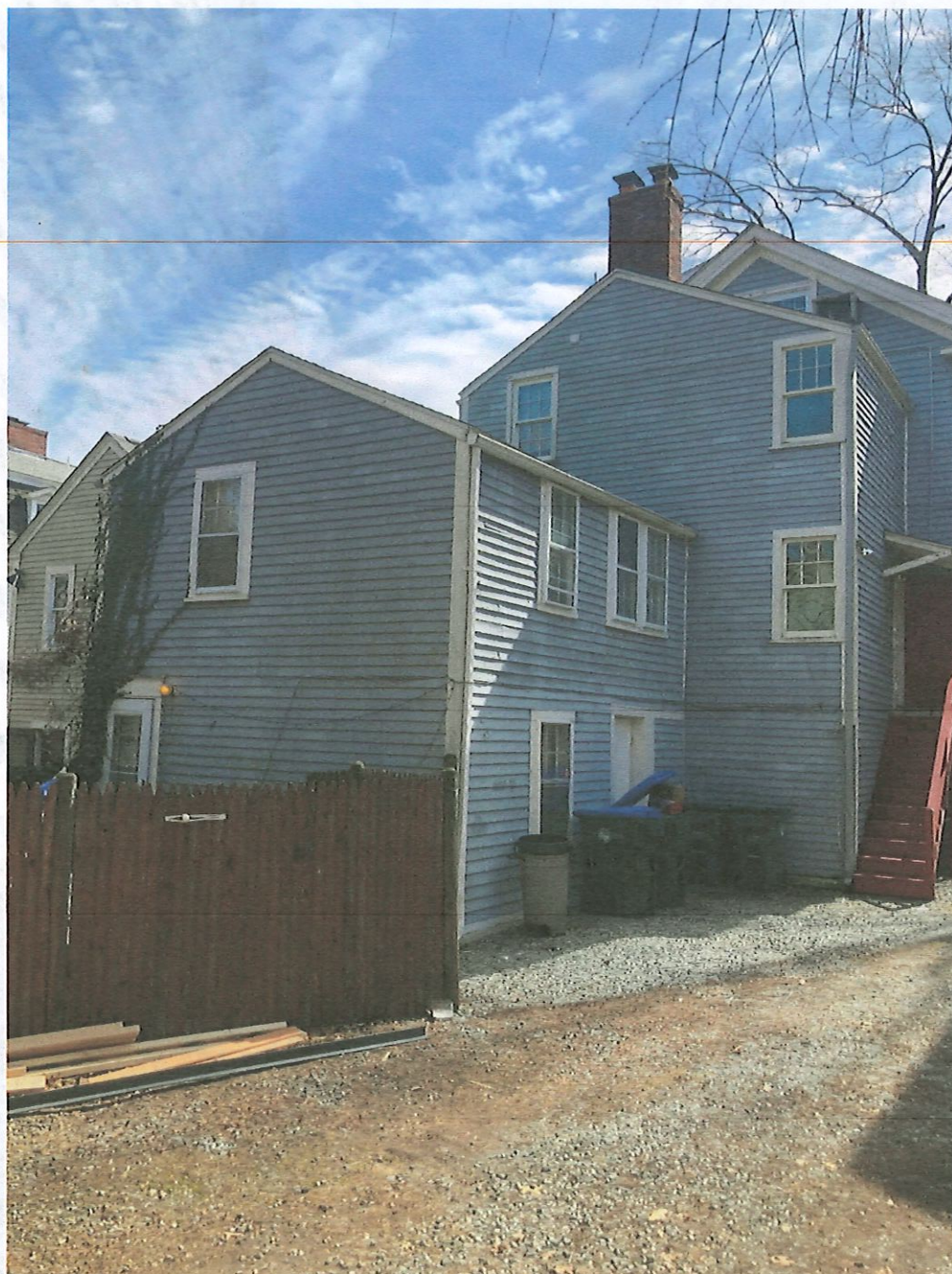
3 - View of rear (north)
