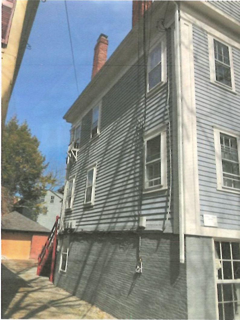
2 - Portion of west wall
