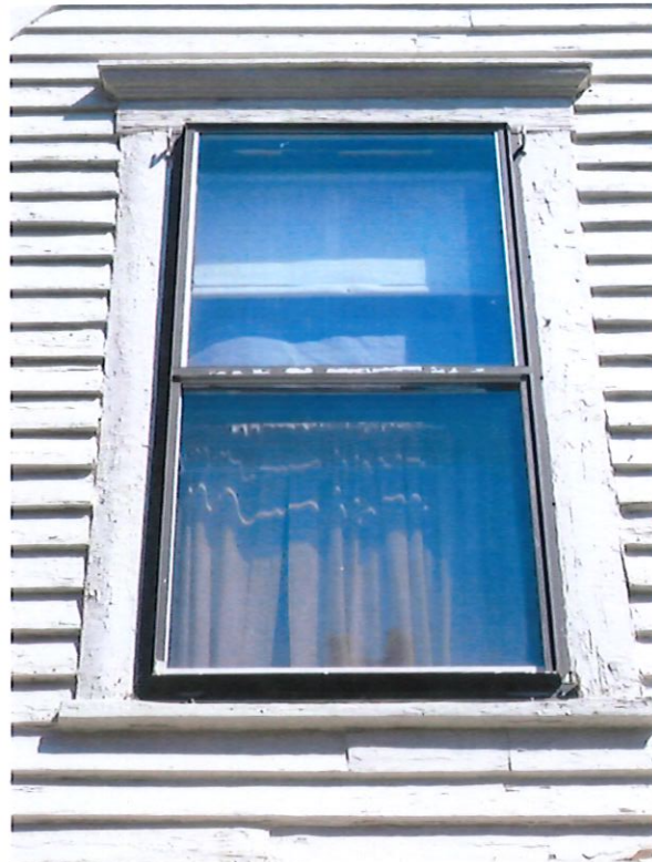
FIGURE 8: South Elevation (Second Floor Window)
