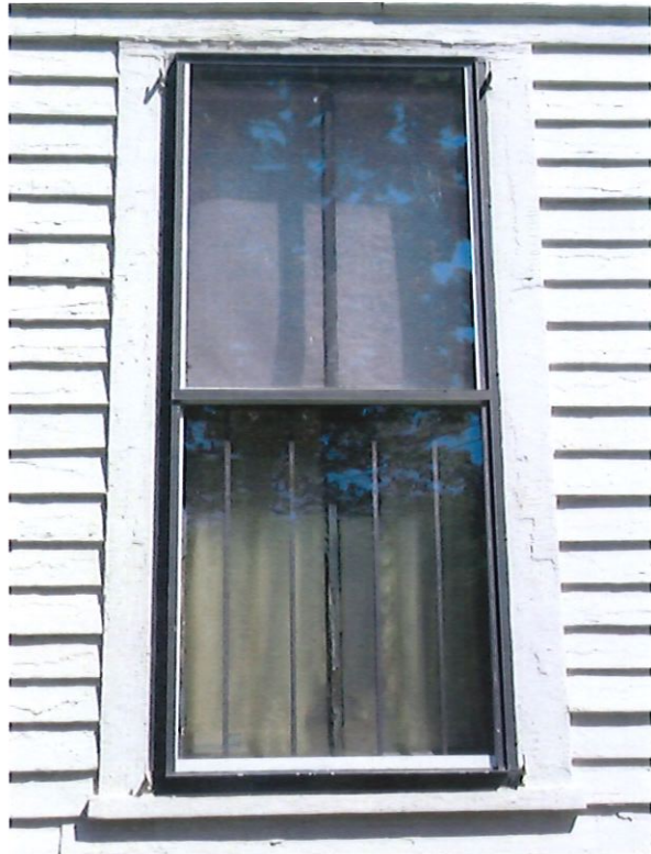
FIGURE 7: South Elevation (First Floor Window)
