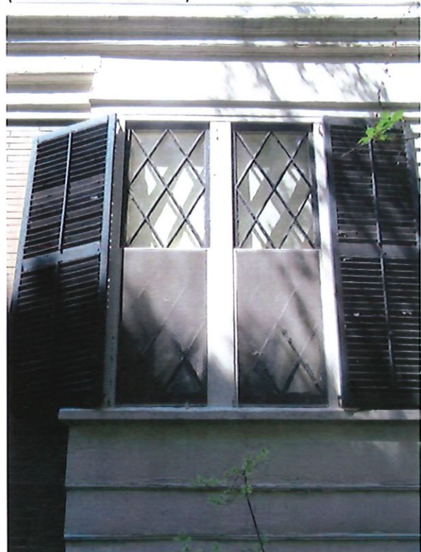
FIGURE 8: East Elevation (First Floor Window)
