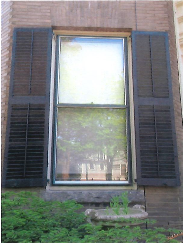
FIGURE 5: North Elevation (First Floor Window)
