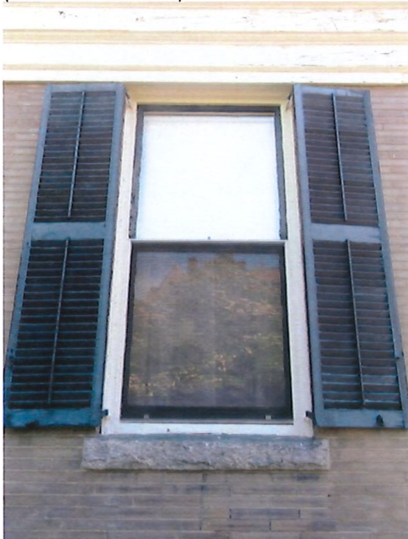
FIGURE 6: West Elevation (First Floor Window)
