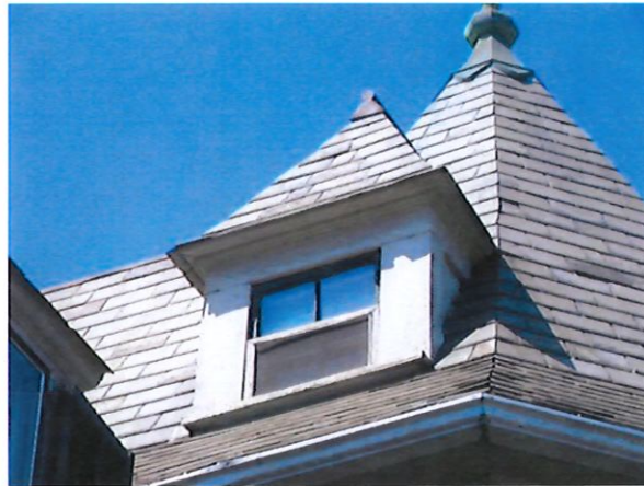
FIGURE 6: North Elevation (Third Floor Window)
