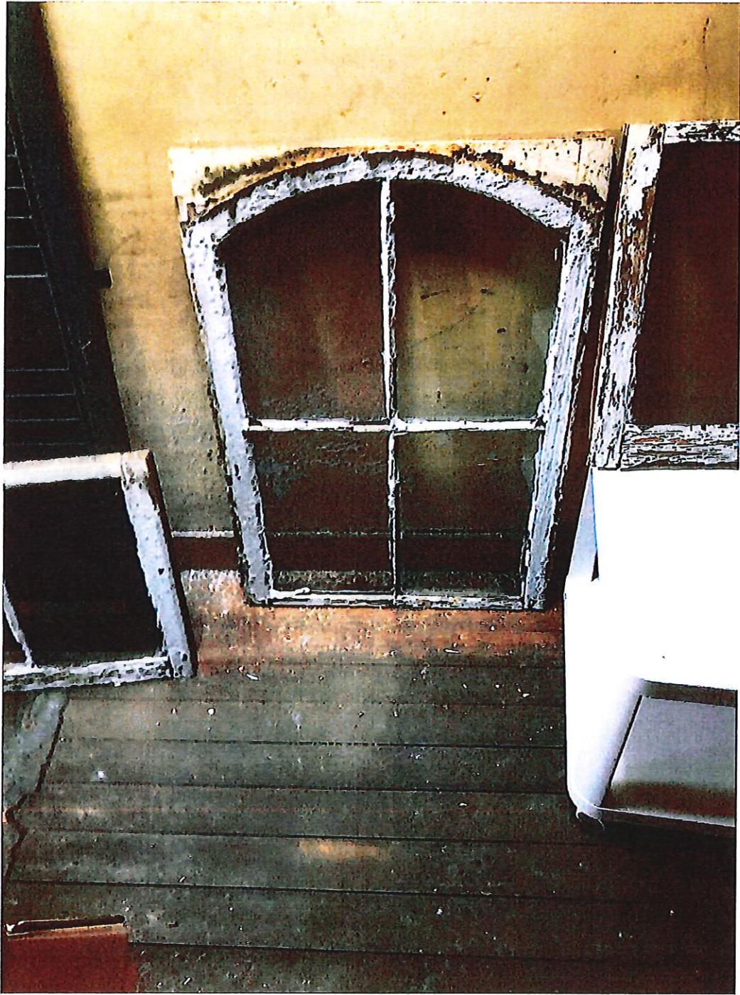
9 - Sashes of "E" units
