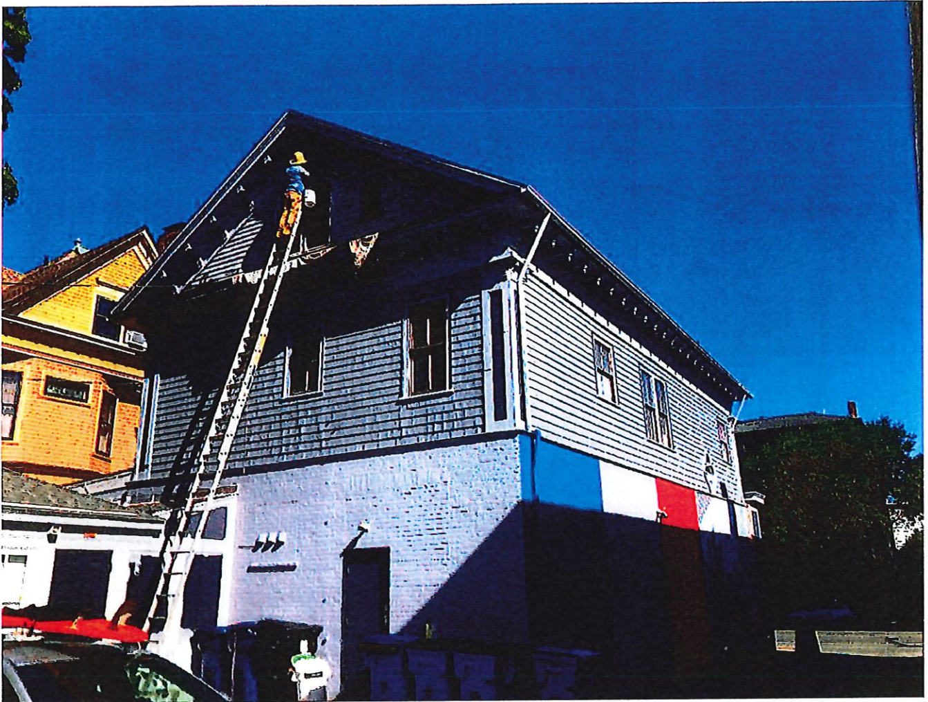
3 - View of SE corner
