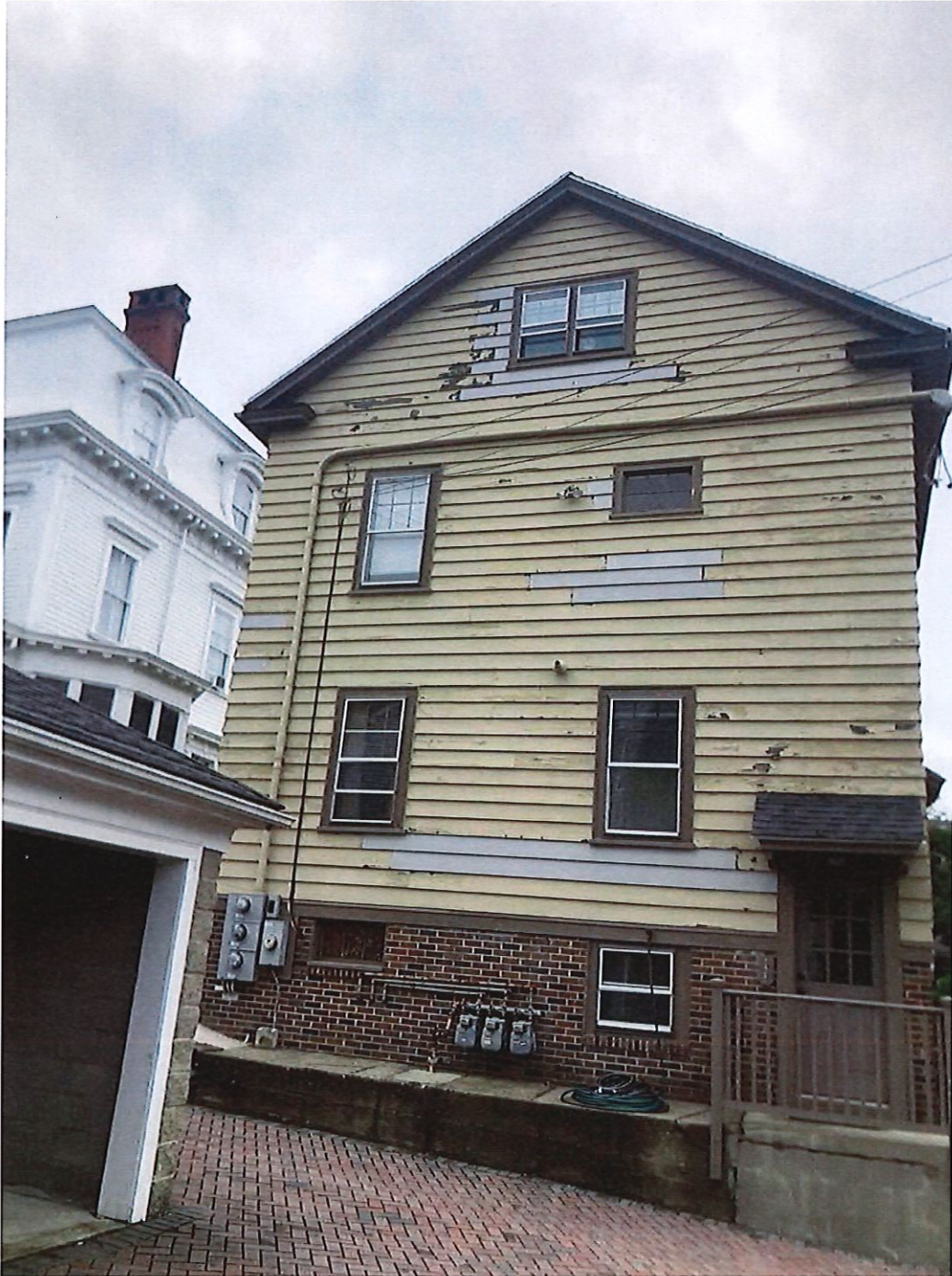
3 - View of rear (east)
