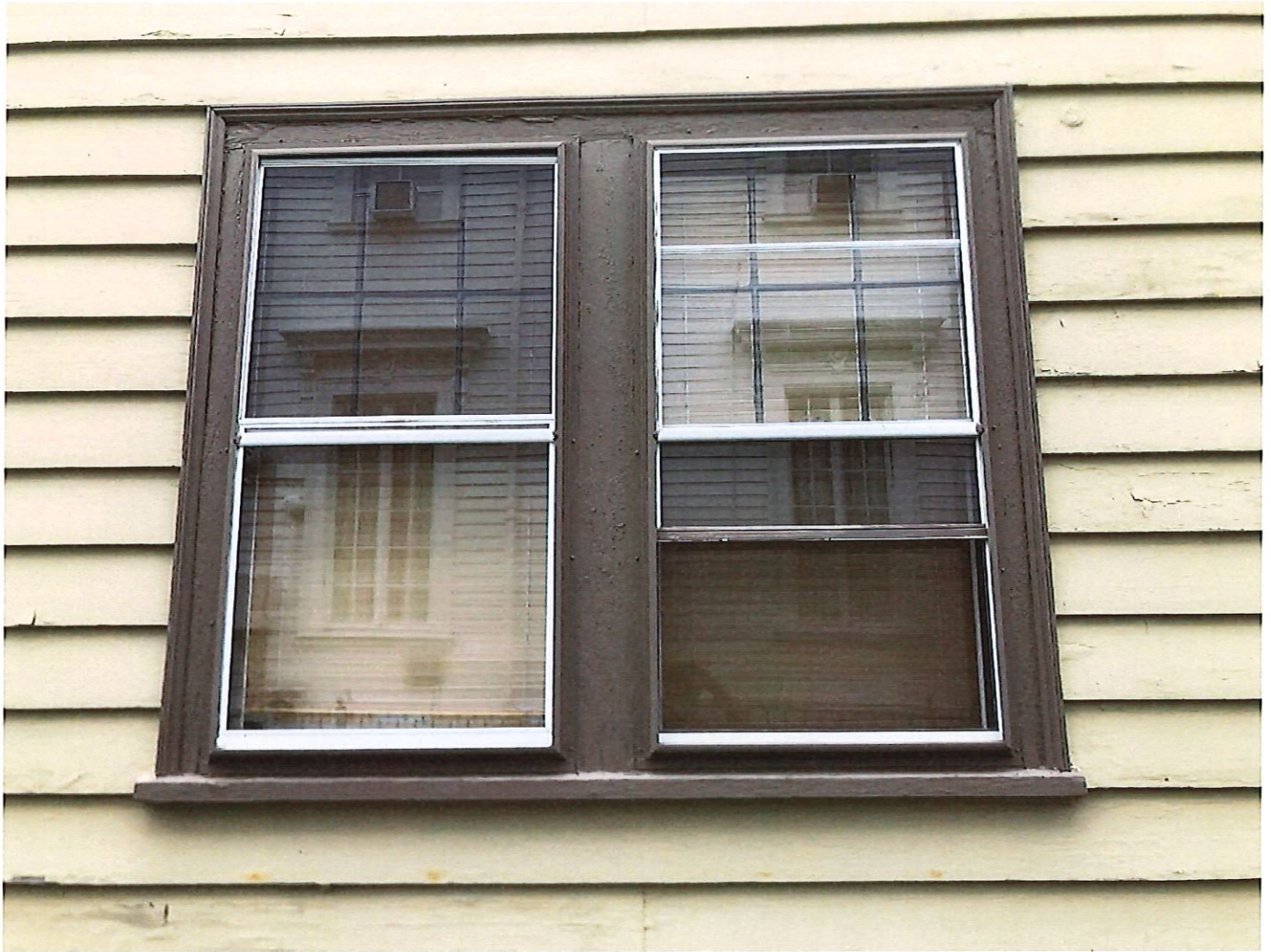
5 - Exterior elevation of units "F"
