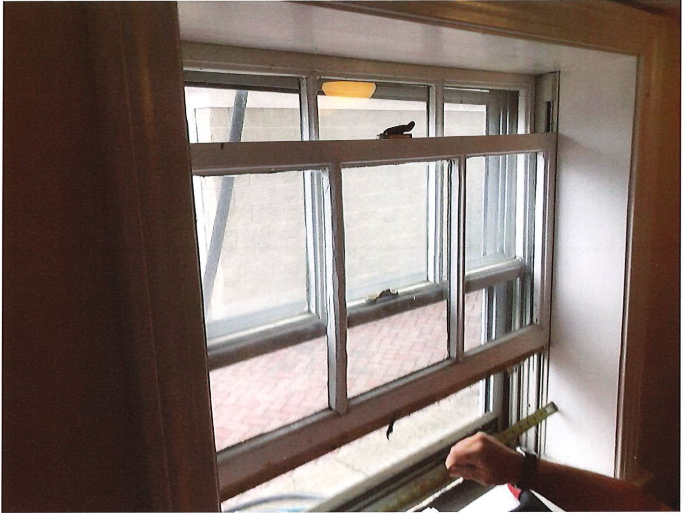
9 - Interior detail at unit "H"
