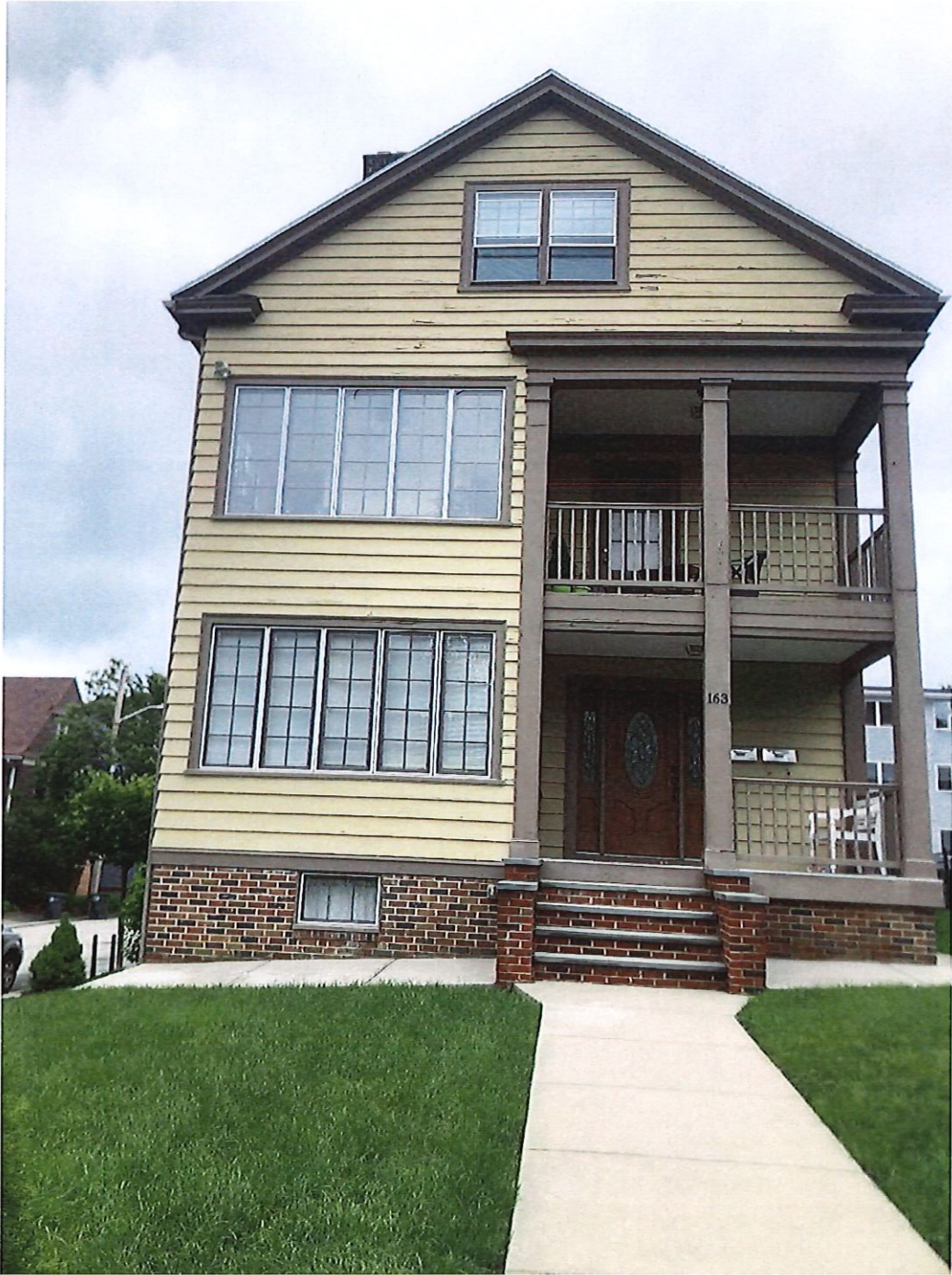
1 - View from Prospect Street (west)
