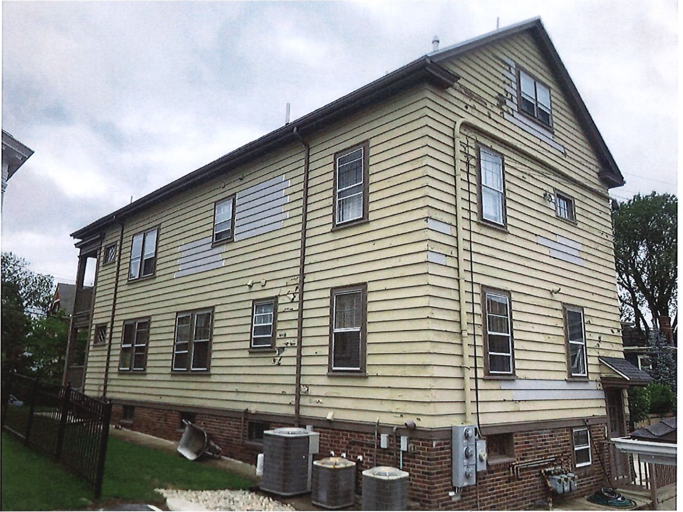
4 - View of SE corner
