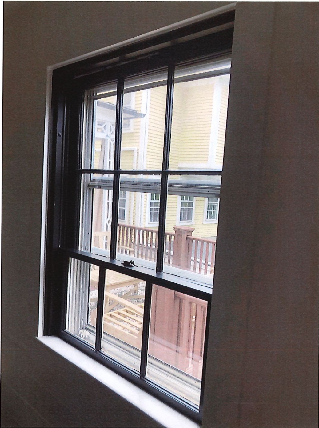
11 - unique "C" units, 6/3, to be replaced
