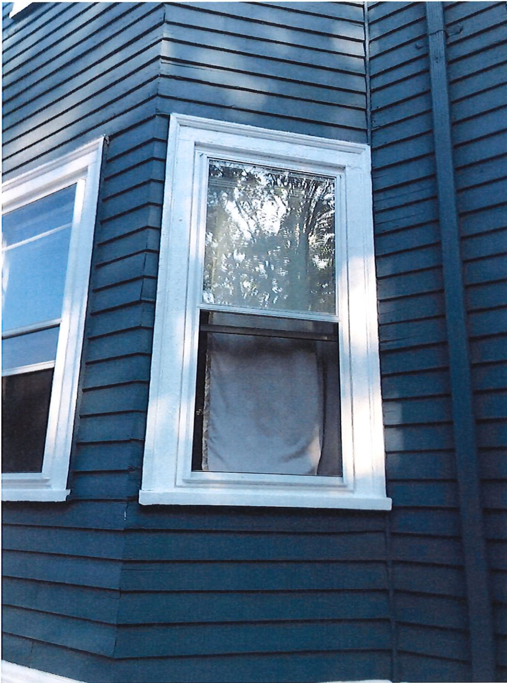
6 - exterior view of window - typical
