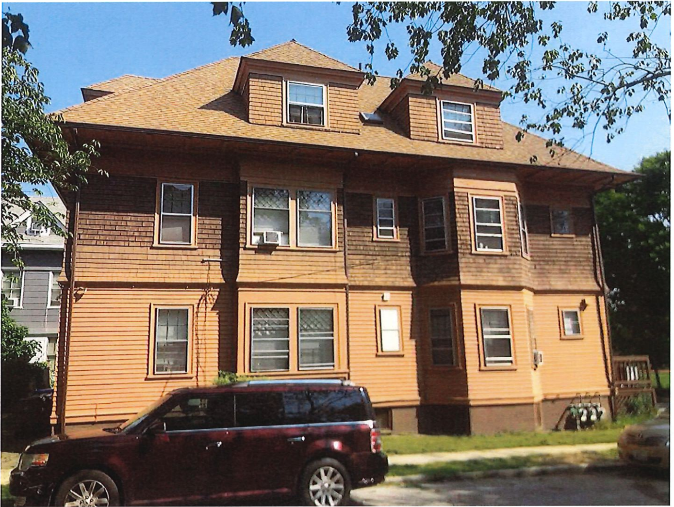
2 - Creighton (south) elevation
