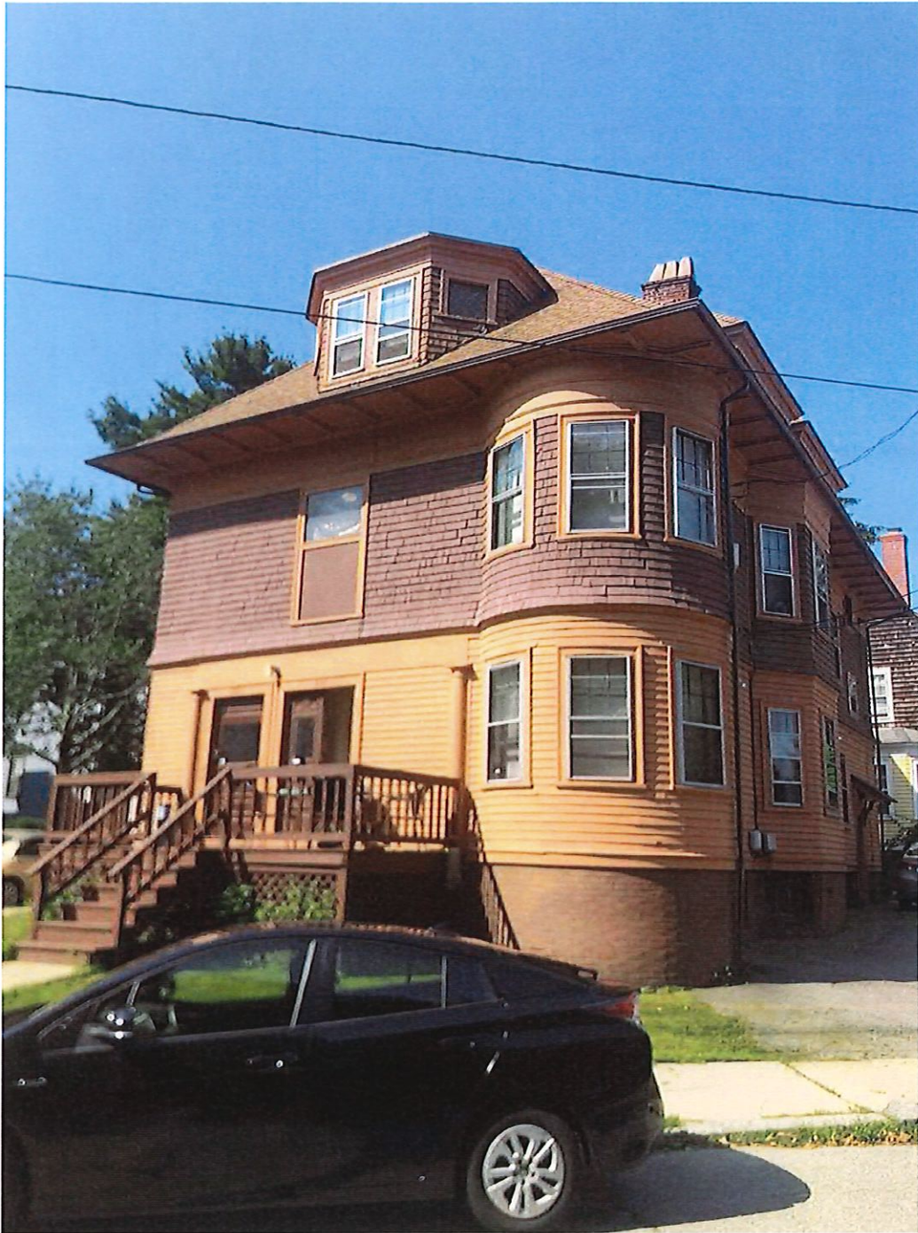
4 - Turret on NE corner
