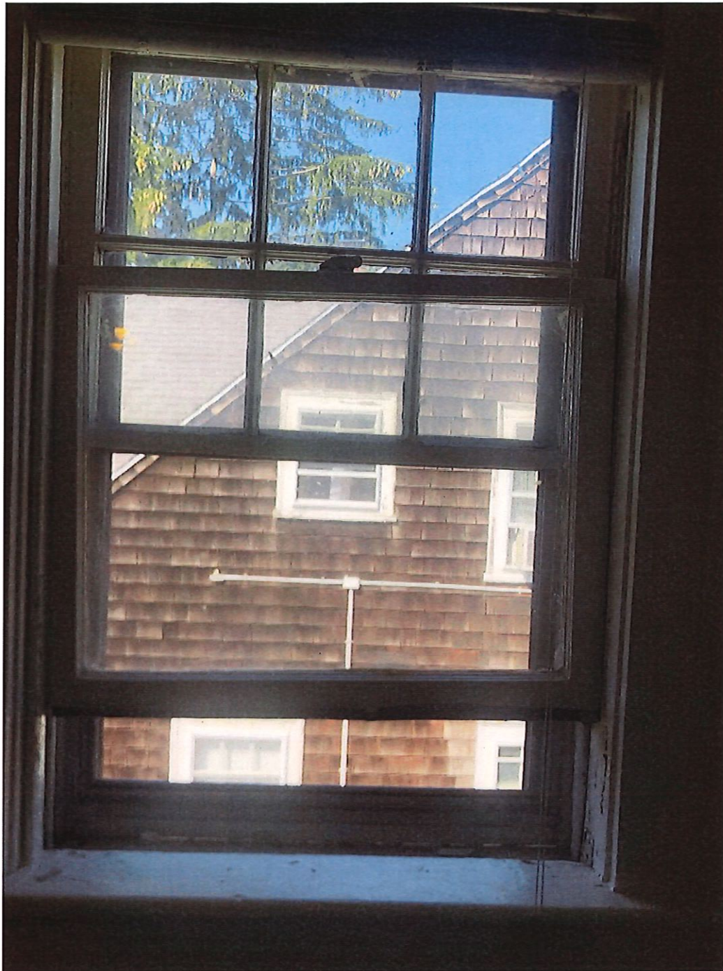
10 - unit "A" from interior
