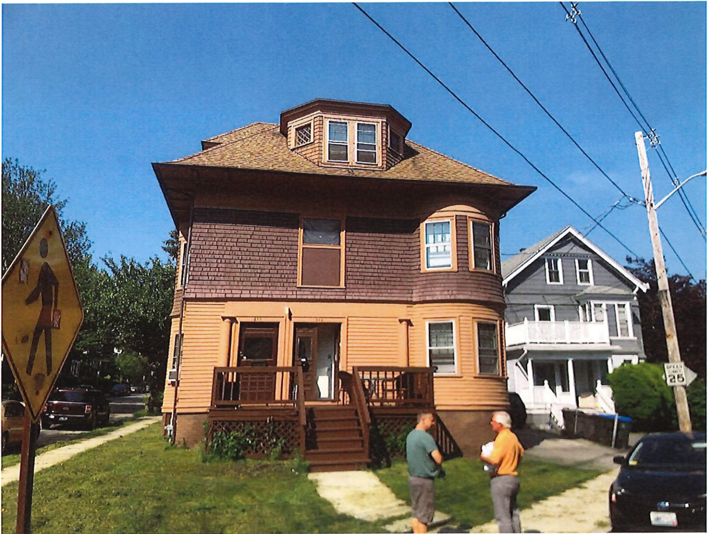
3 - Brown Street (east) elevation
