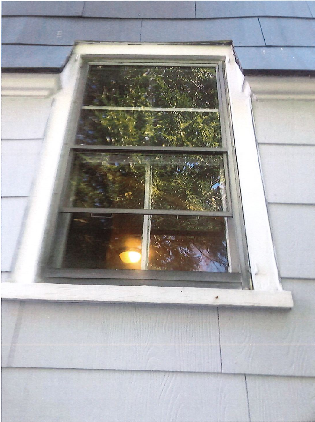
6 - Exterior window detail
