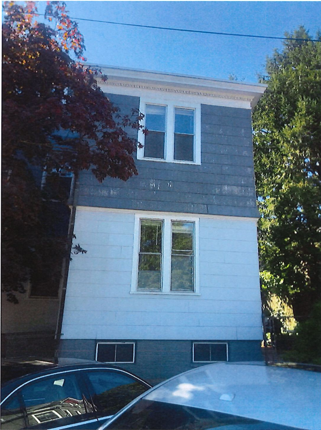
3- detail of north wall projection - windows "H"
