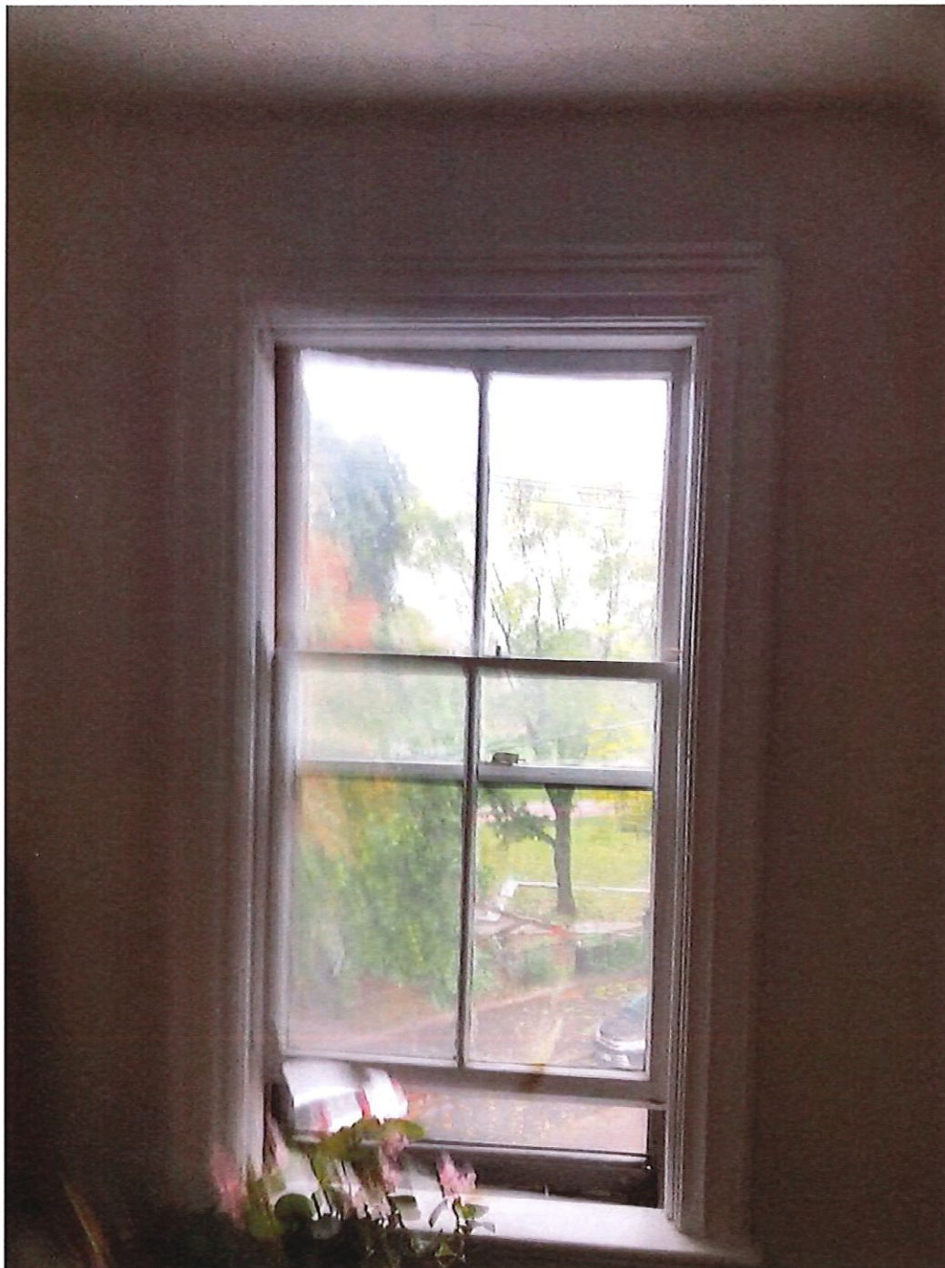
7 - interior view of window
