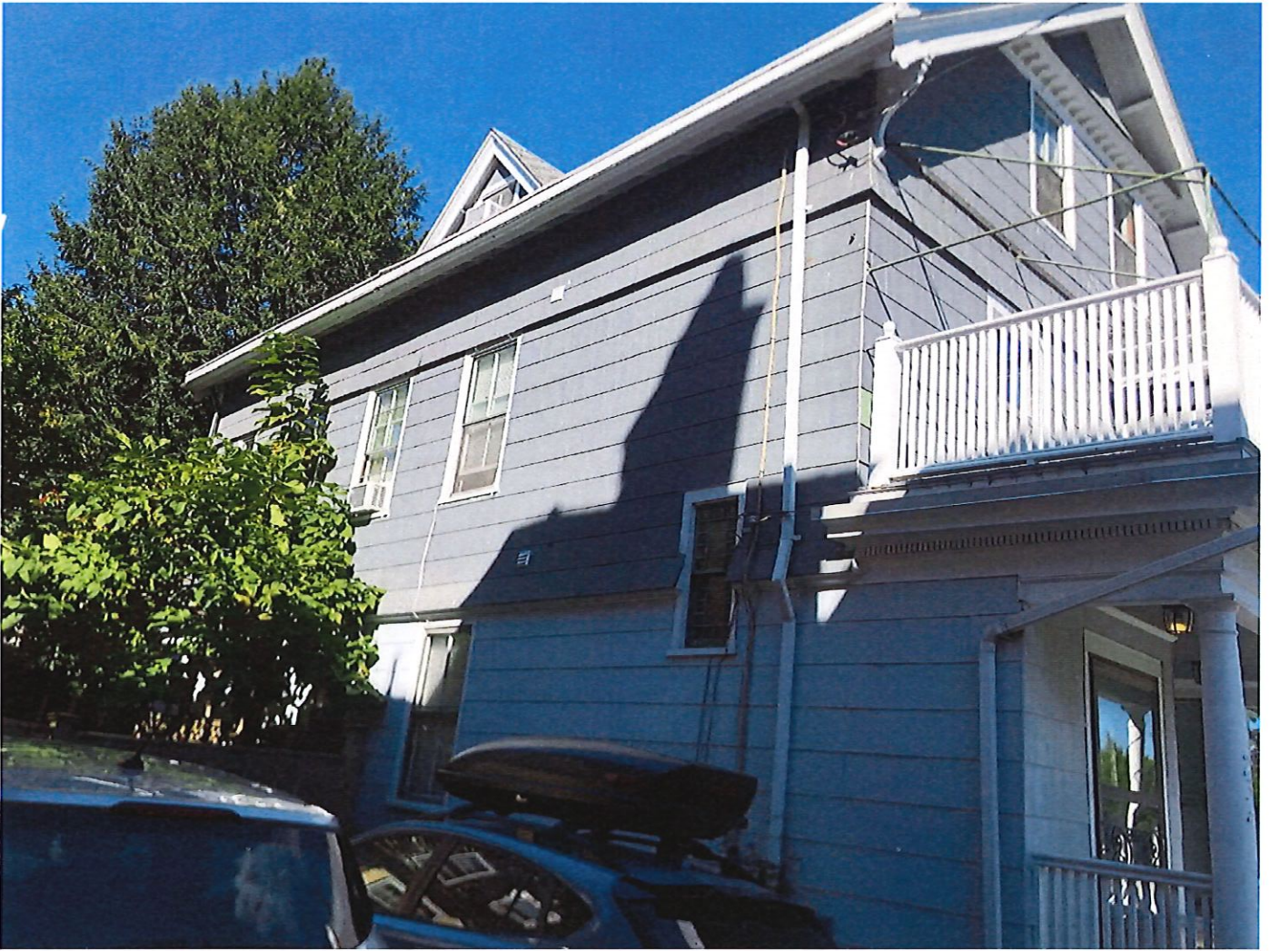
2 - Portion of south elevation
