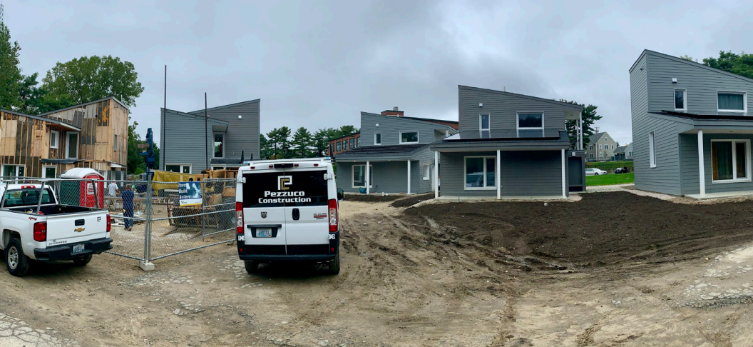
Sheridan Small Homes by ONE Neighborhood Builders.
