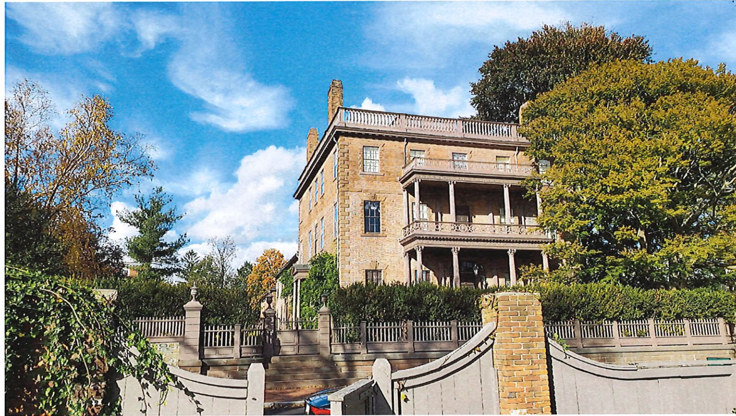
66 WILLIAMS STREET - CORLISS / CARRINGTON HOUSE
